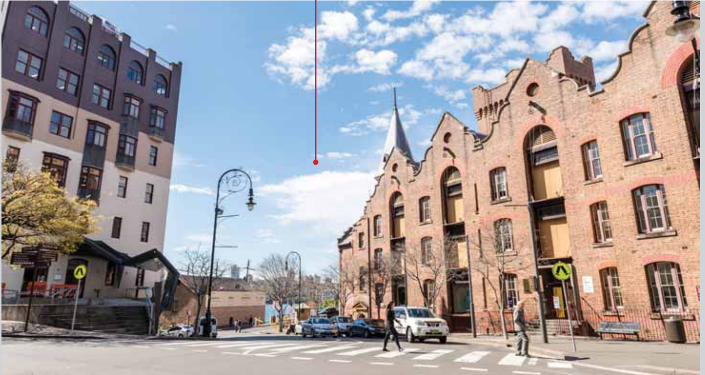
EXISTING View from George Street Photograph provided by Virtual Ideas
