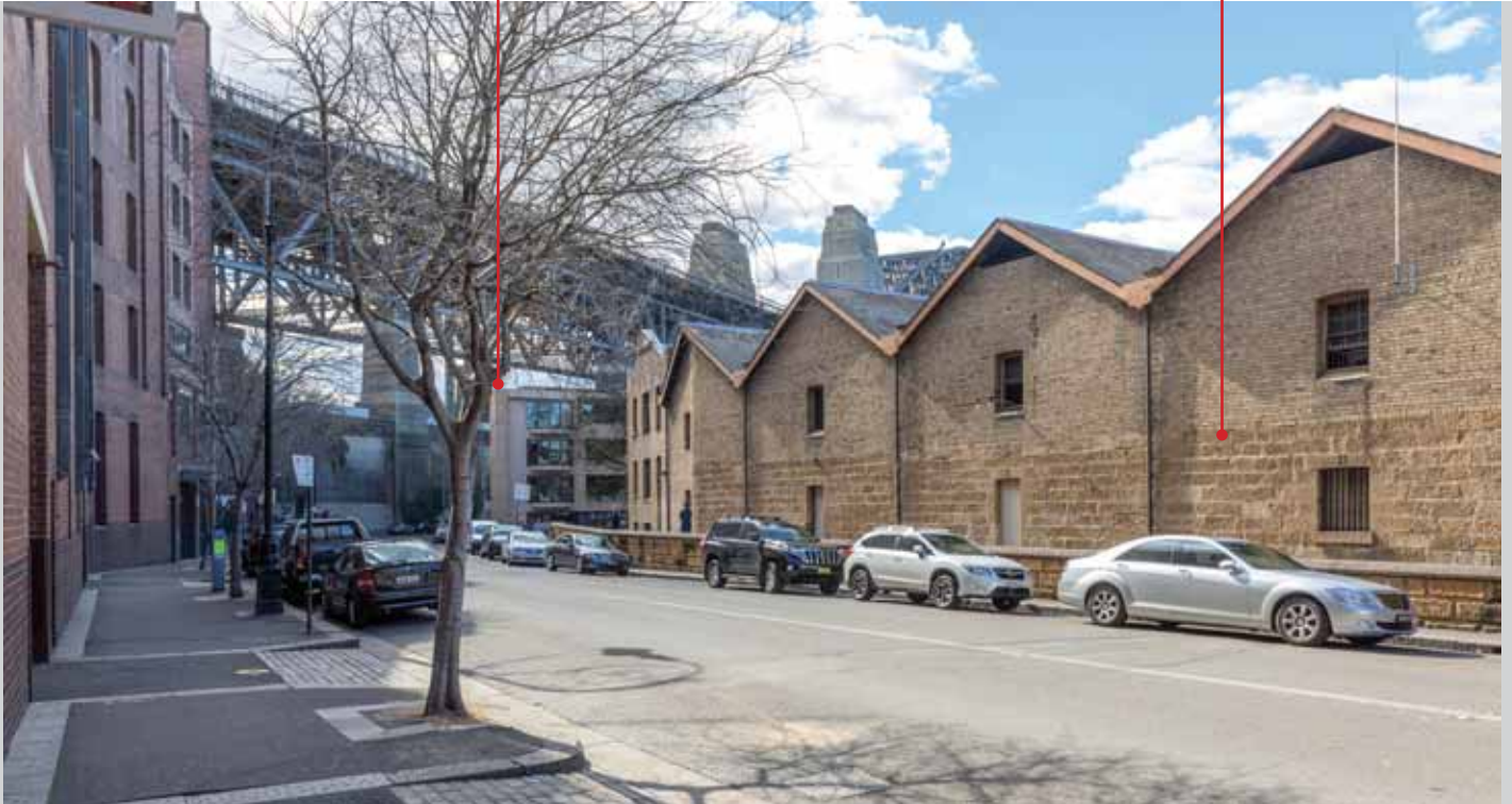
EXISTING Hickson Road View from Bay 6 Photograph provided by Virtual Ideas
