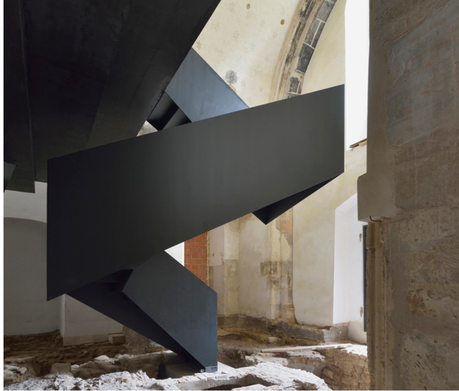
Steel fabricated stair finished with warm grey tone MIO paint
