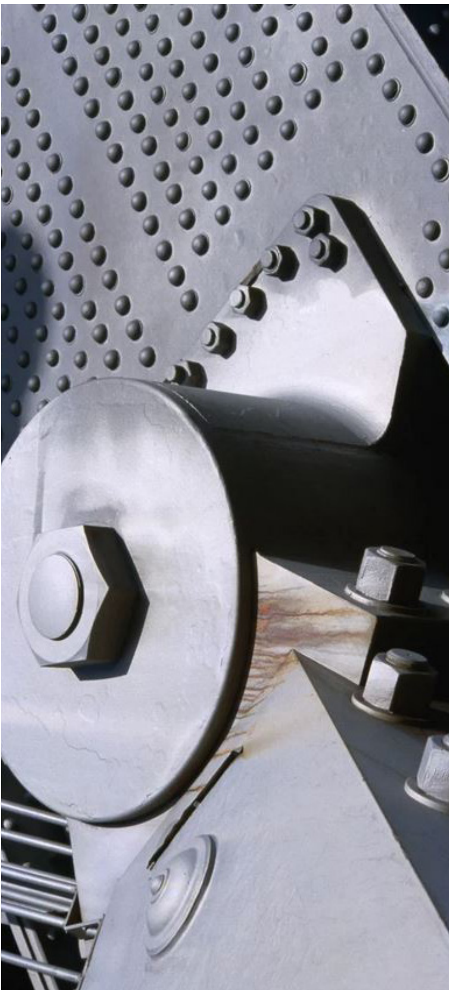
HARBOUR BRIDGE STEEL CONNECTION
