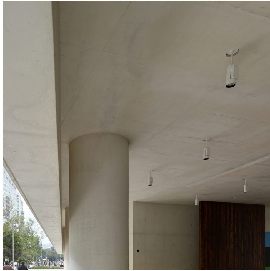
CONC1 Off form concrete Class 2 with warm coloured aggregates consistent with Campbell's Stores
