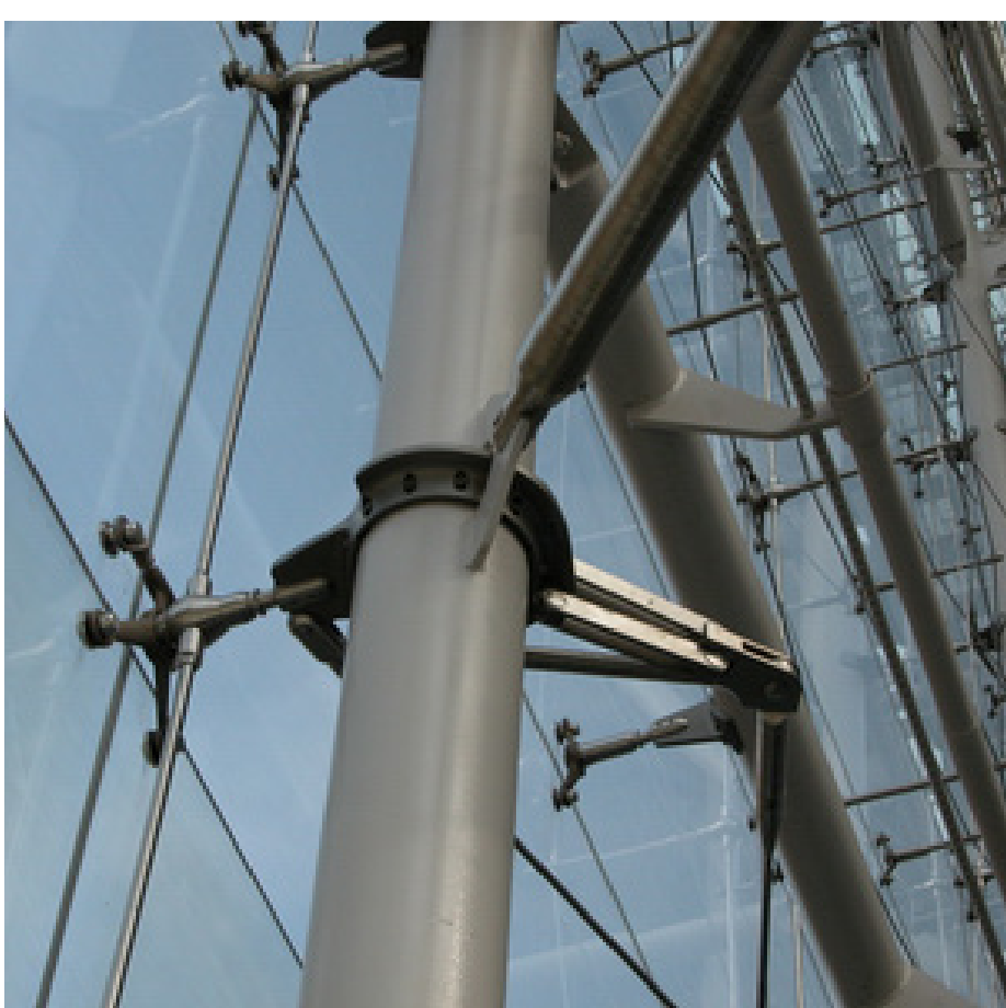
New steel structure- Facade components & Fixings Finished with warm grey MIO paint
