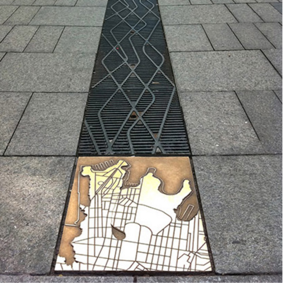
Metal feature drain with interpretive elements
