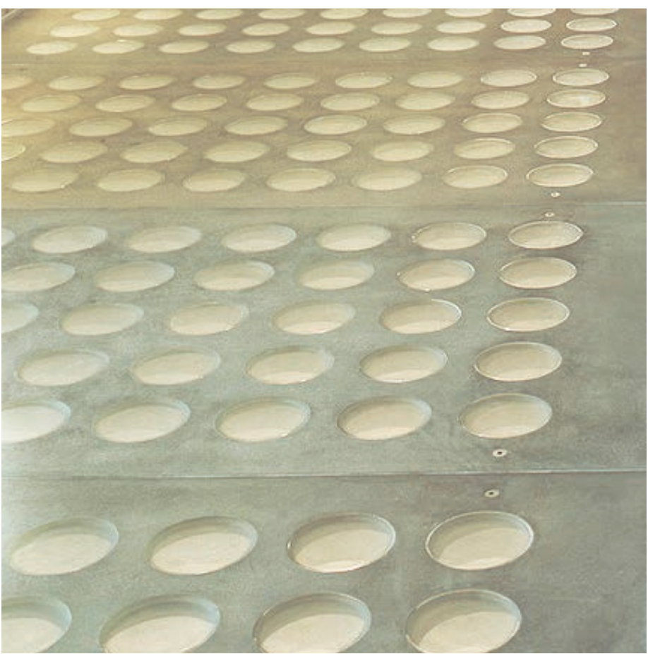
PC High quality finish (e.g. honed, polished) perforated precast concrete with glass infills or cast insitu (min. class 2 finish) - warm tone consistent with Campbell's Stores.
