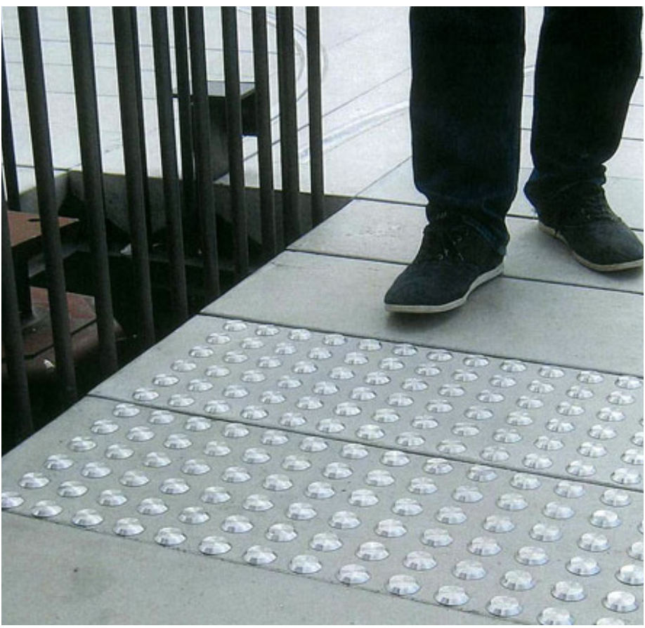
PAVE4 Abrasive blasted exfoliated precast concrete sleepers
