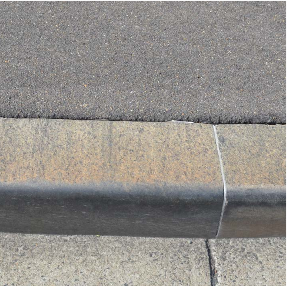
PAVE5 Stone kerbs as per CoS requirements
