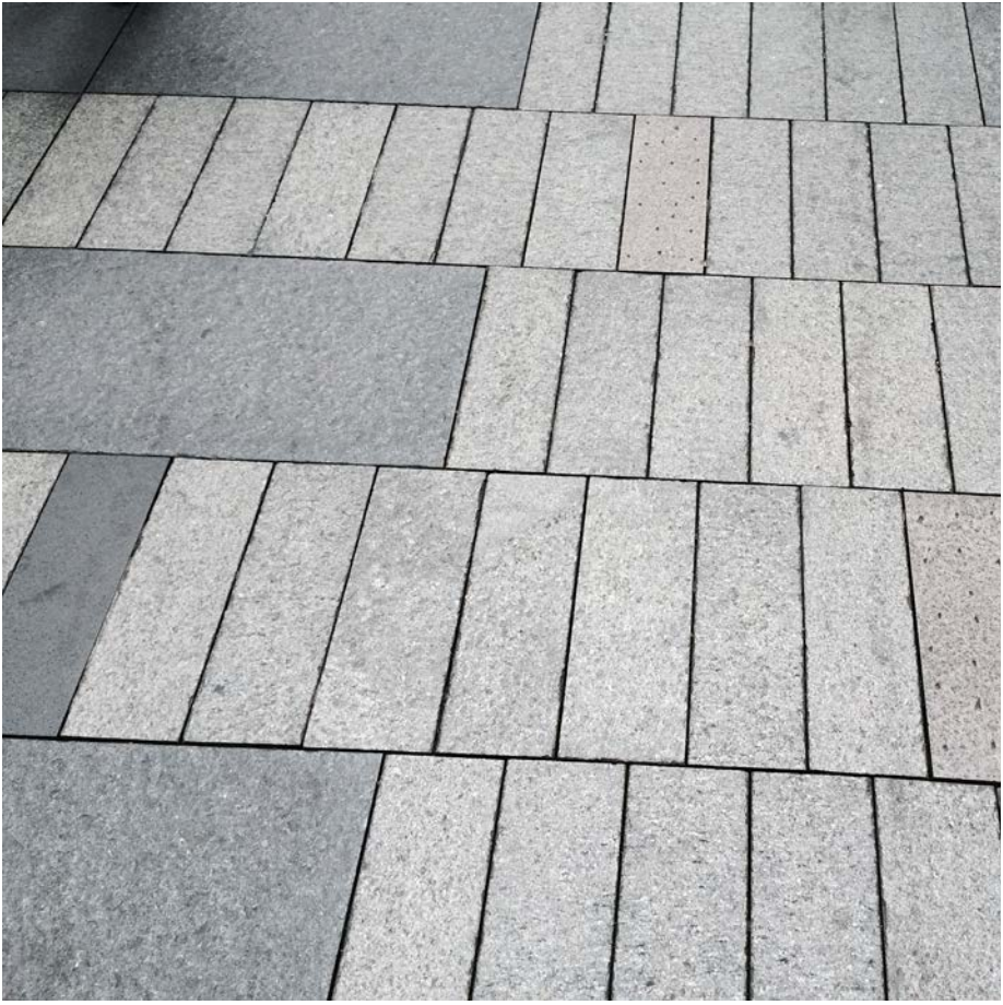
PAVE1 Stone pavers to match C.o.S finishes
