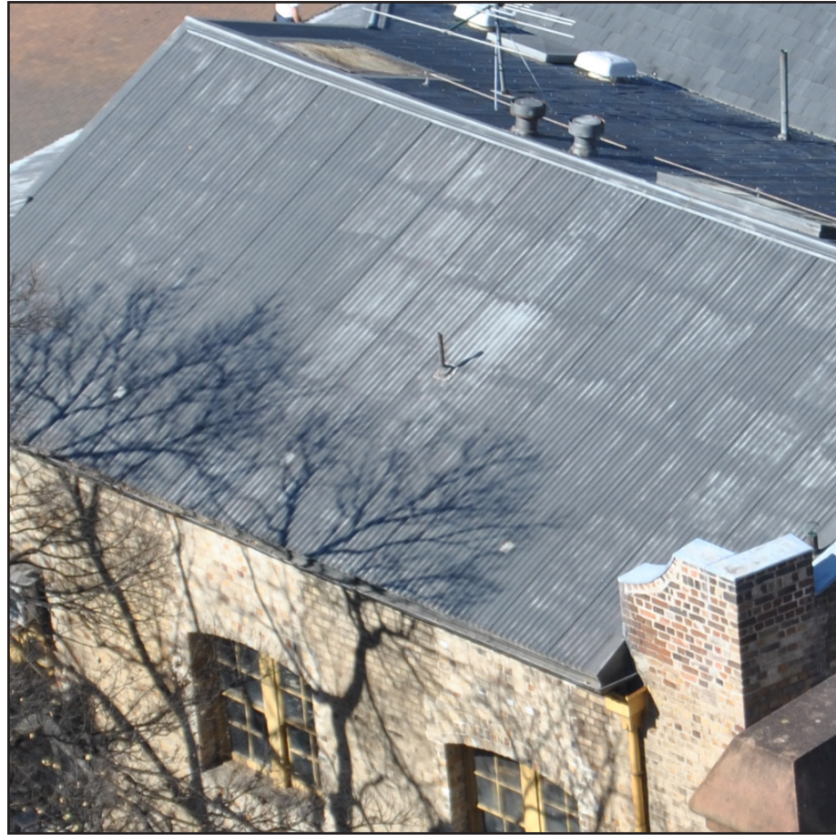
MS Metal roof sheet to match existing
