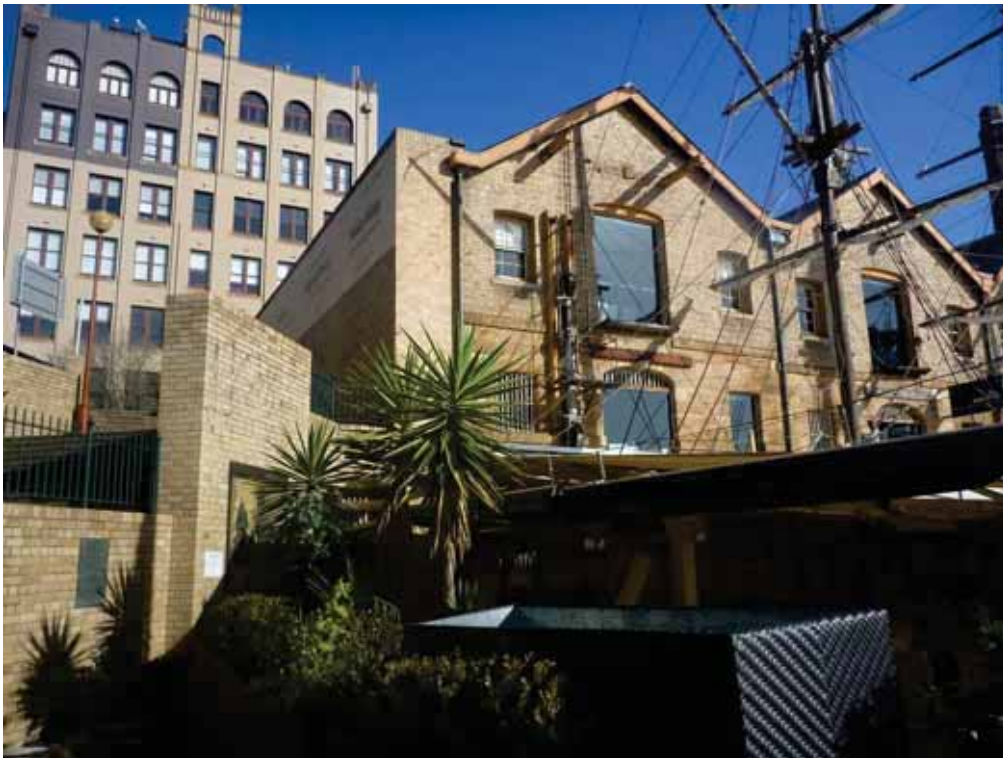
Figure 7.3 East facing view showing the southern extent of Campbell's Stores and new brick addition, with the stairs situated in the former location of the stores' southern bay.
