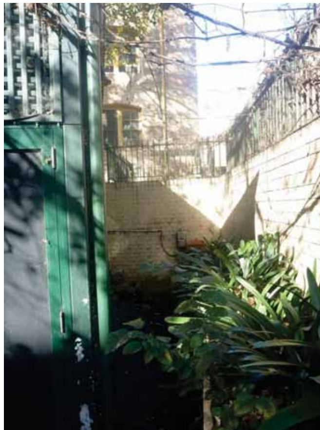
Figure 7.9 South facing view showing the western retaining wall between Hickson Road and the lower area to the north of the stores.
