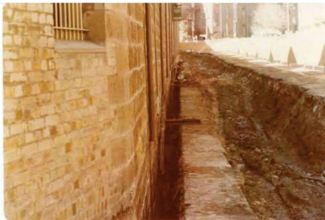
Figure 8.6 Excavation for the western service tunnel in the 1970s (SHFA in GML 2014: 91)
