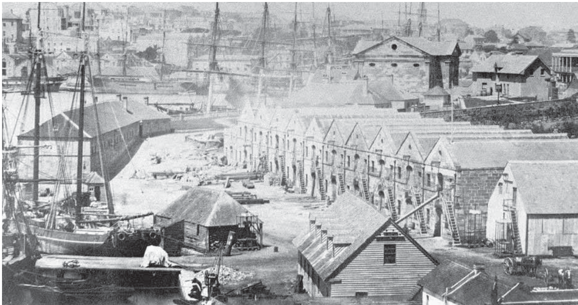
Figure 5.3 Photograph showing construction of the eleventh Campbell's Stores bay, c.1860s (SHR, Campbell's Stores Listing)
