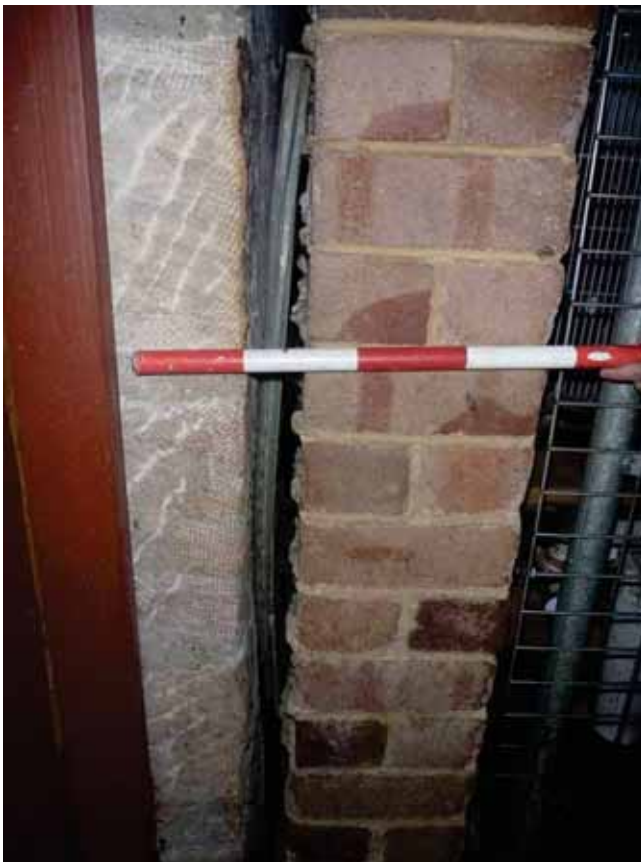
Figure 7.5 South facing view within the western service tunnel showing the western sandstone wall of Campbell's Stores abutting the brick retaining wall addition.
