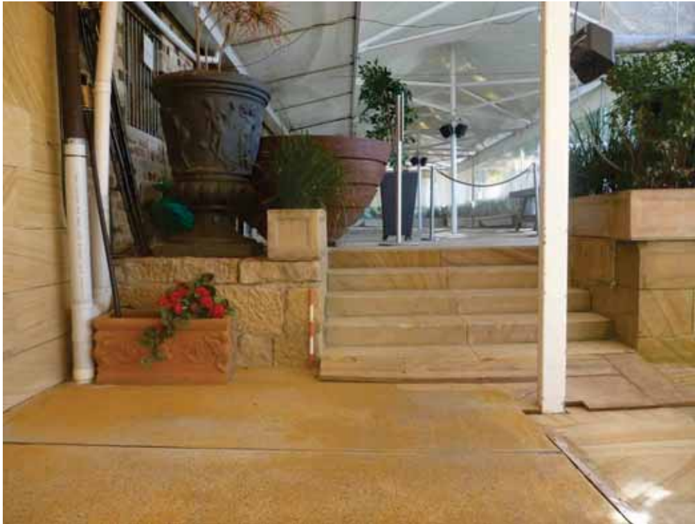
Figure 7.8 North facing view showing the relative level of the Bay 11 seating area.
