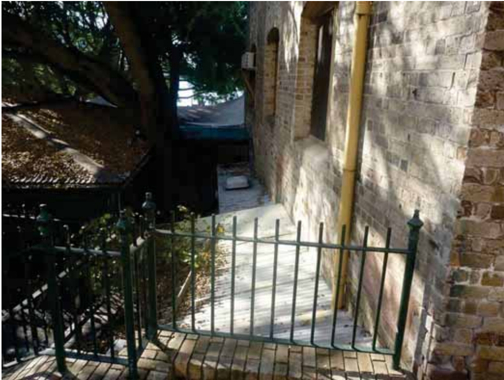
Figure 7.6 East facing view showing the northern face of the Campbell's Stores and the attached superficial structural elements which mark the end of the service tunnel.
