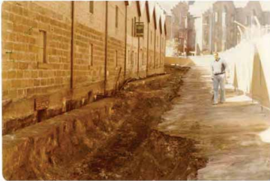
Figure 8.7 Excavation for the western service tunnel in the 1970s (SHFA in GML 2014: 91)
