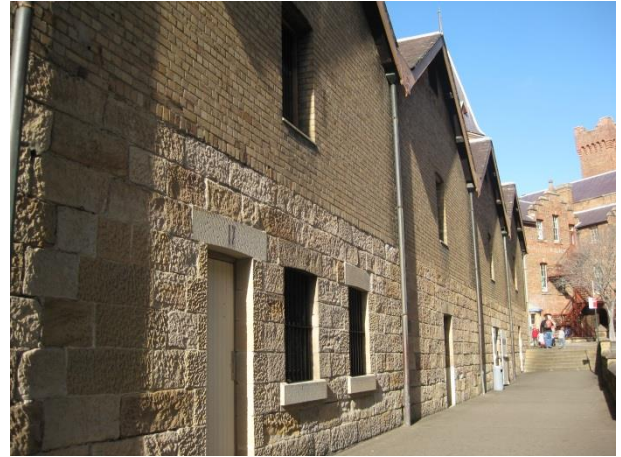
PICTURE 2 – HICKSON ROAD FRONTAGE AND FOOTPATH (WITH TUNNEL BELOW)
