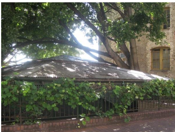
PICTURE 5 – EXISTING STANDALONE BUILDING TO NORTH OF CAMPBELL'S STORES BUILDING
