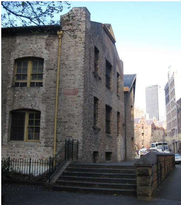
PICTURE 3 – NORTH WESTERN CORNER OF BUILDING ON HICKSON ROAD
