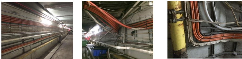
Figure 3.3 – Consumer mains and submains on cable trays
