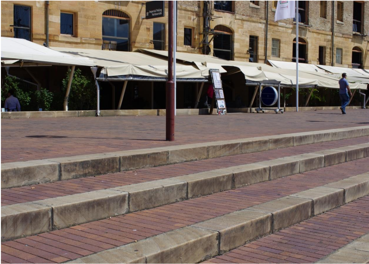
Figure 2: Existing Campbell's Cove Promenade looking toward Campbell's Stores from waterfront
