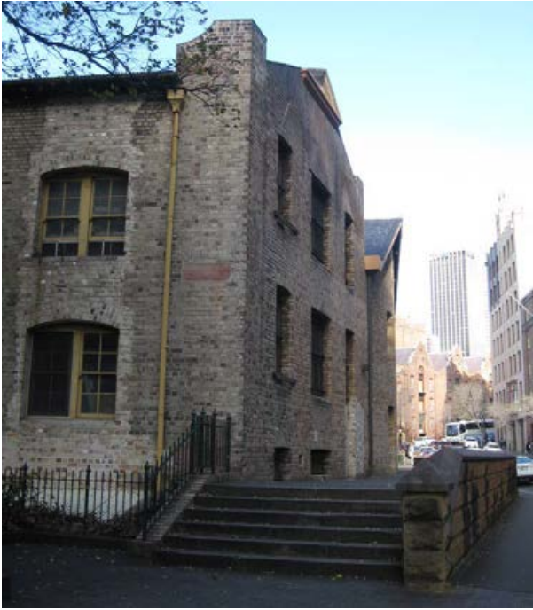
PICTURE 3 – NORTH WESTERN CORNER OF BUILDING ON HICKSON ROAD
