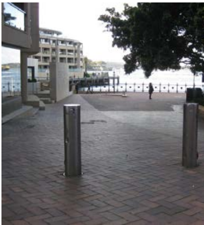
PICTURE 12 – ACCESS FROM HICKSON ROAD ON NORTHERN SIDE OF CAMPBELL'S STORES
