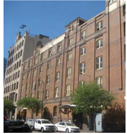
— PICTURE 14 – METCALFE BOND STORES ON WESTERN SIDE OF HICKSON ROAD
