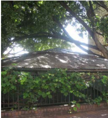
PICTURE 5 – EXISTING STANDALONE BUILDING TO NORTH OF CAMPBELL'S STORES BUILDING
