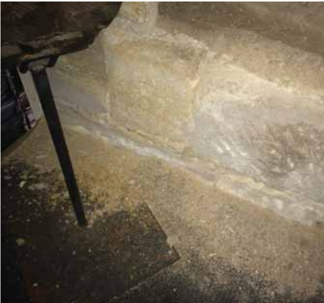
Figure 2.2.2 Example of section of wall deteriorating due to rising damp, including spalling.
