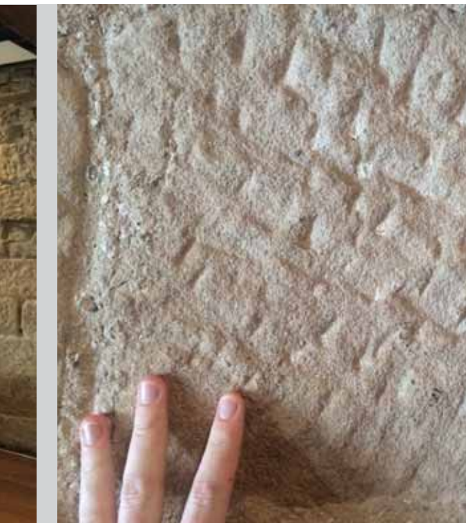
Figure 2.2.3 Example of existing sandstone with convict-hewn markings
