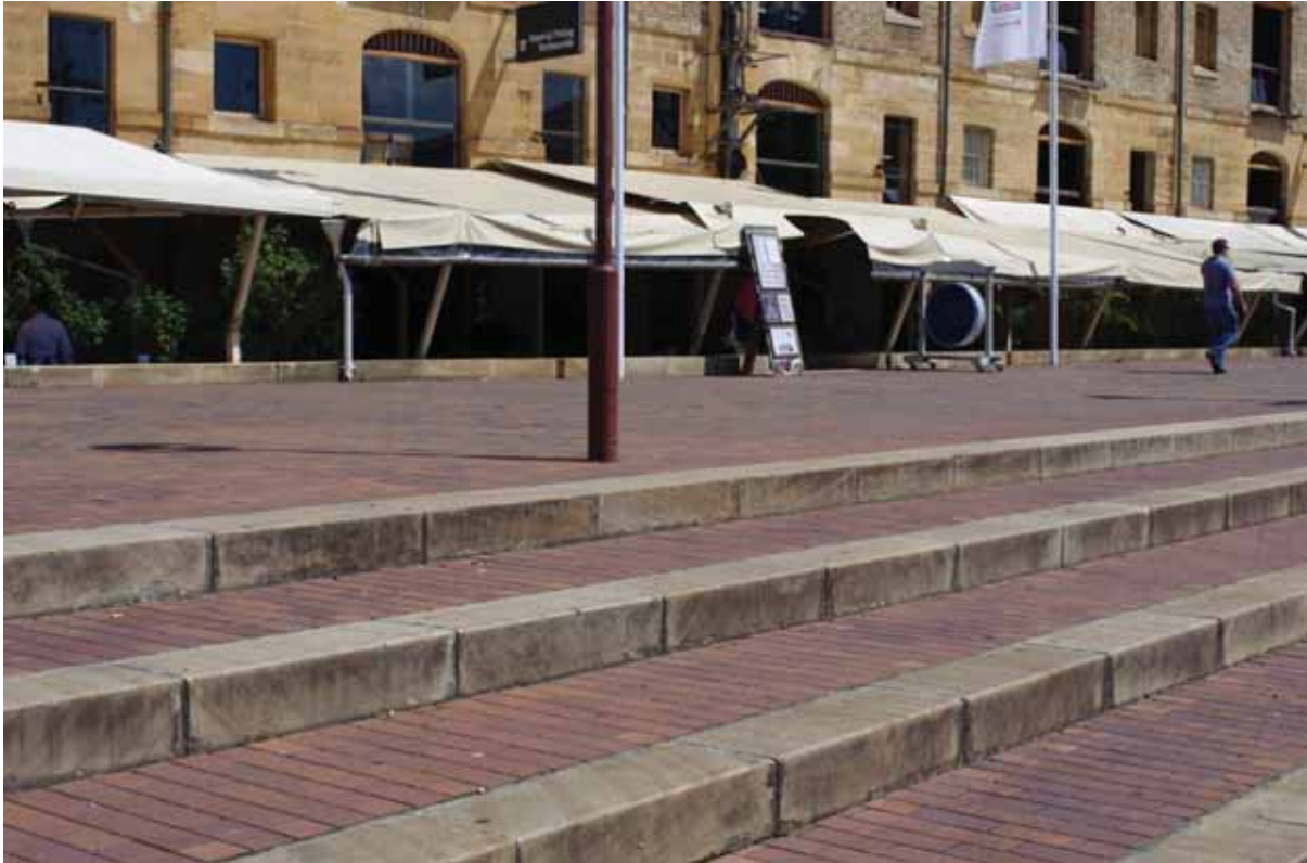
Existing Campbell's Cove Promenade looking toward Campbell's Stores from waterfront
