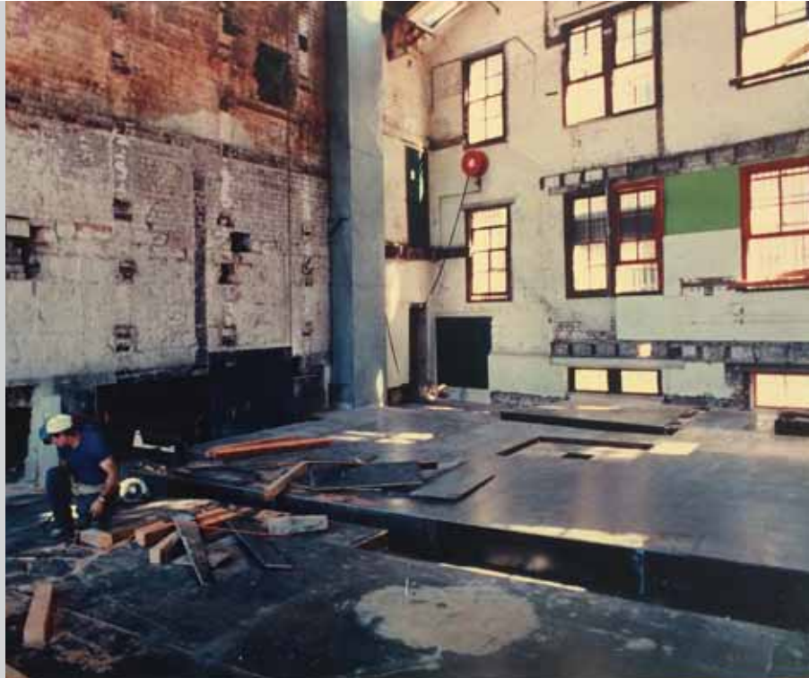
Figure 2.4.4 Campbell's Stores Bay 11, with all floors removed
