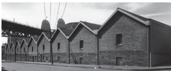
Figure 2.4.6 Campbell's Stores 1970 showing windows and new doors
