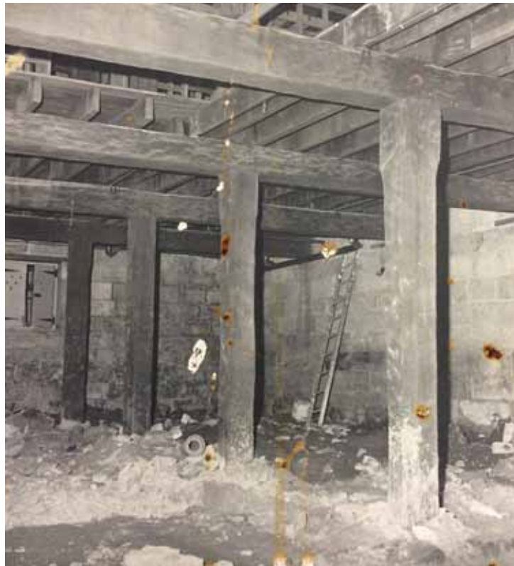
Figure 2.4.3 Campbell's Stores ground floor, with flooring removed
