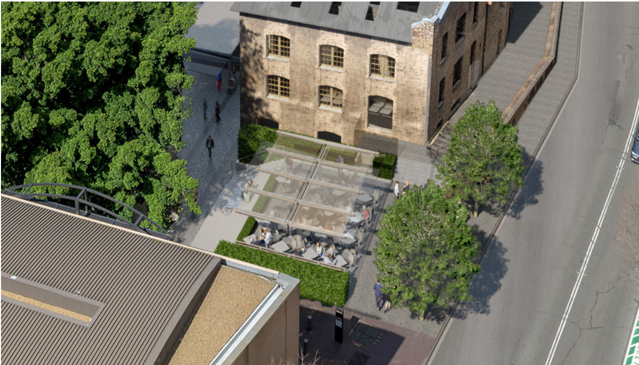
Figure 8. Birds eye view of northern terrace demonstrating multiple access points and open sight lines (source JPW)
