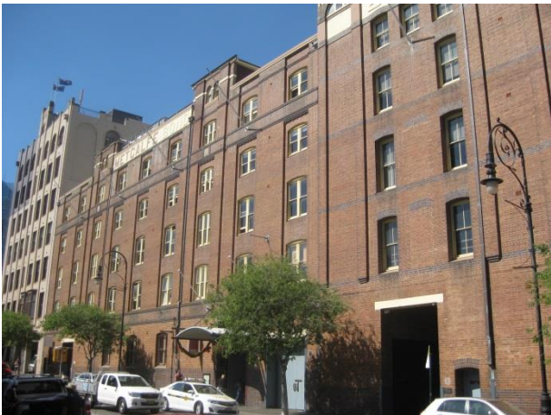
PICTURE 8 – METCALFE BOND STORES ON WESTERN SIDE OF HICKSON ROAD
