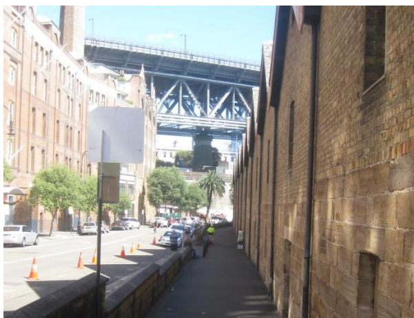
PICTURE 2 – HICKSON ROAD FRONTAGE AND FOOTPATH (WITH TUNNEL BELOW)
