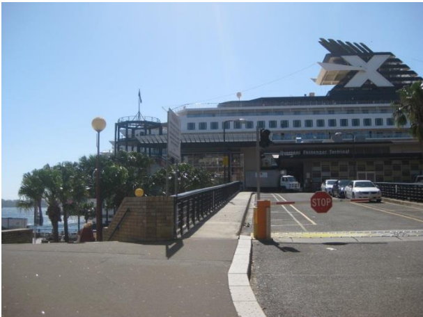
PICTURE 6 – OVERSEAS PASSENGER TERMINAL ACCESS DRIVEWAY (ABOVE LOADING DOCK)
