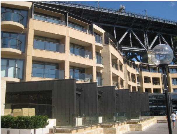
PICTURE 7 – PARK HYATT SYDNEY AND FORESHORE PROMENADE TO NORTH OF CAMPBELL'S STORES
