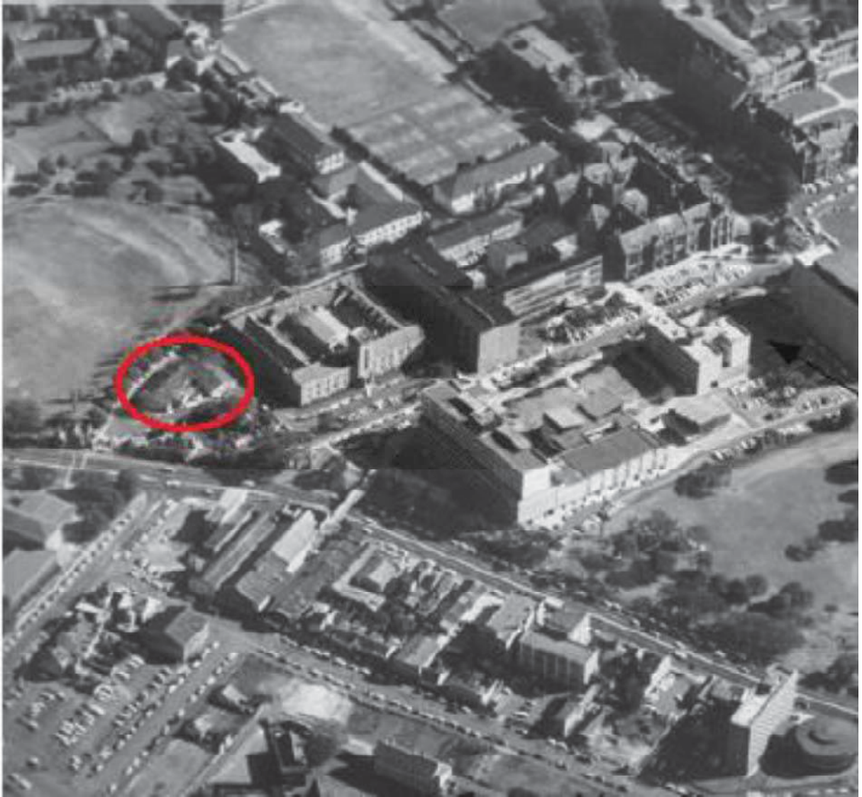
Figure 2.11 1969 orthographic aerial showing a v-shaped building in the proposed Administration Building area north west of City Road and open ground where the Carslaw Building currently stands. (Source: JoMcD 2005 with GML additions 2015 33 )
