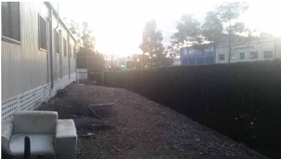
Figure 3.5 Example of steep battering of slopes adjacent to Parramatta Road, fill overlying in foreground (Source: GML 2015)
