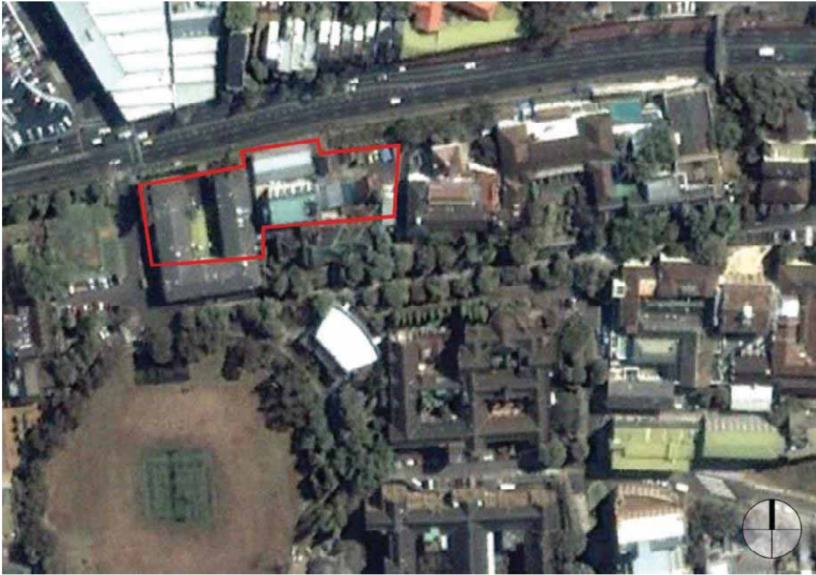
Figure 2.12 Detail of the site showing the Ross Street Building prior to demolition in 2010 aerial photo. (Source: Google Earth with GML Additions).
