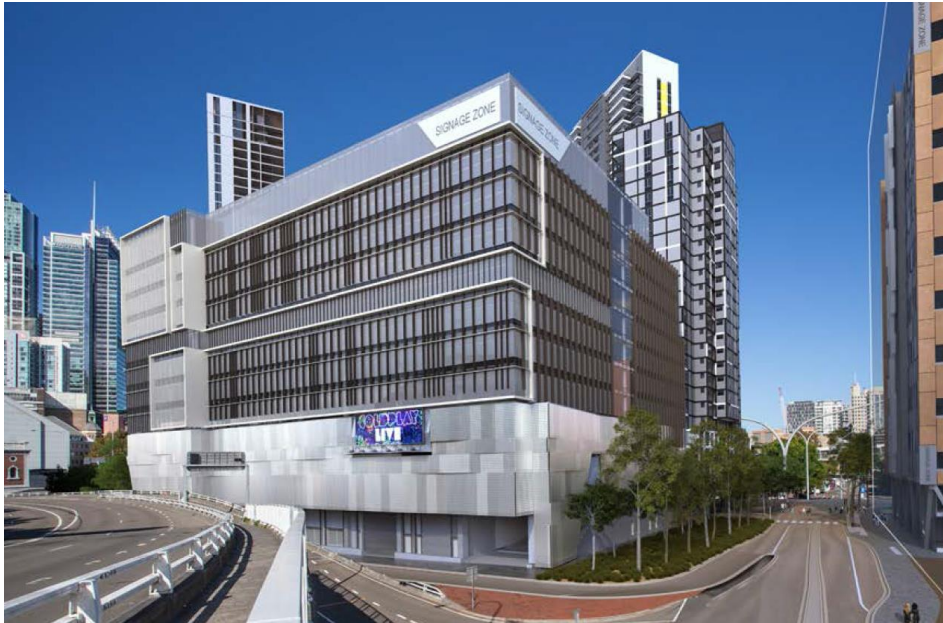
Figure 3 – Approved North-West Plot Building and its Digital Sign
