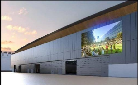
Southern façade of ICC Sydney Exhibition – the Event Deck (E-02)
