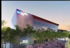
Static sign – Eastern façade of ICC Sydney Theatre (T-09)
