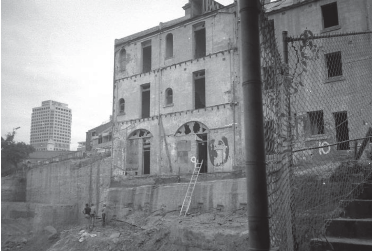
FIGURE 19 – EXCAVATION OF CAMBRIDGE STREET FOR THE CONSTRUCTION OF HARRINGTON COURT, 1980S
