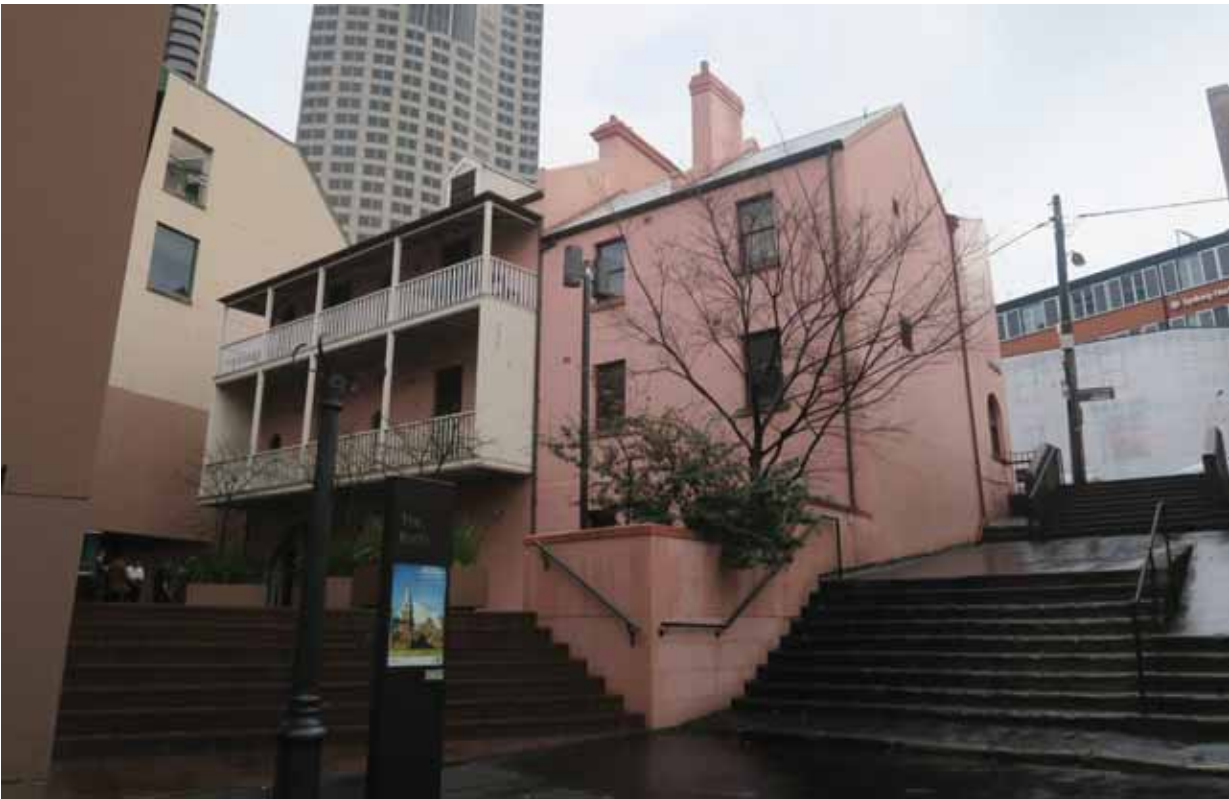
FIGURE 3 – REAR OF BAKER'S TERRACE AND STAIRS LEADING TO CAMBRIDGE STREET ON THE LEFT AND TO CUMBERLAND PLACE ON THE RIGHT.
