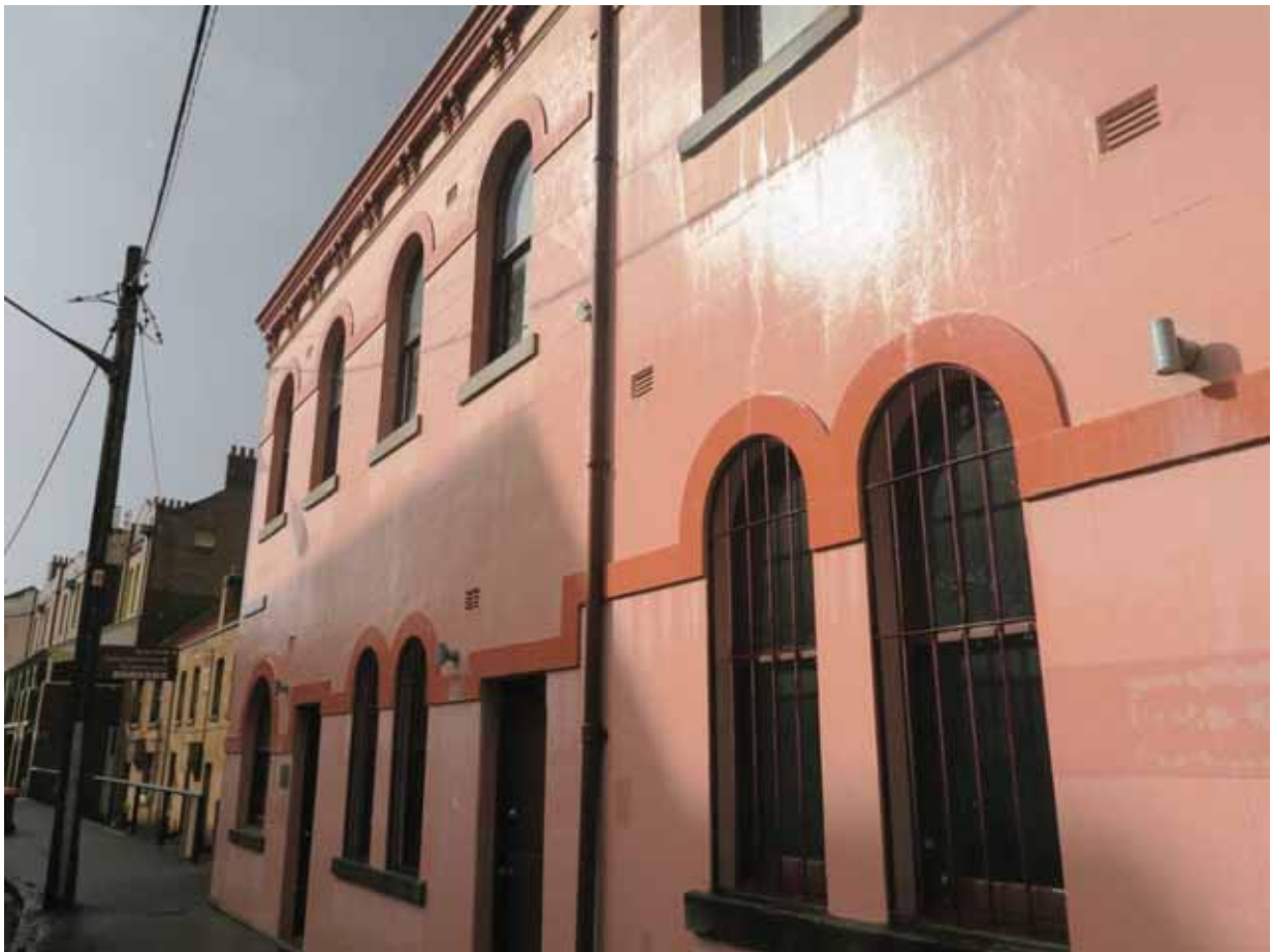
FIGURE 2 – GLOUCESTER STREET FRONTAGE OF BAKER'S TERRACE
