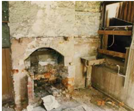
PICTURE 14 – BASEMENT OF NO. 68 SOURCE: FUTUREPAST CMP 2006
