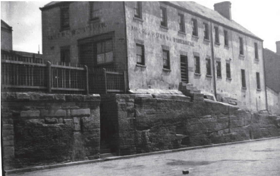
FIGURE 14 – THE SAILORS RETURN TO THE NORTH OF STUDY AREA ON HARRINGTON STREET AROUND 1915. THE STAIRS TO CUMBERLAND PLACE CAN BE SEEN CUT INTO THE BEDROCK AND THE SANDSTONE WALL ON THE LEFT REMAINS IN THE STREET TODAY.
