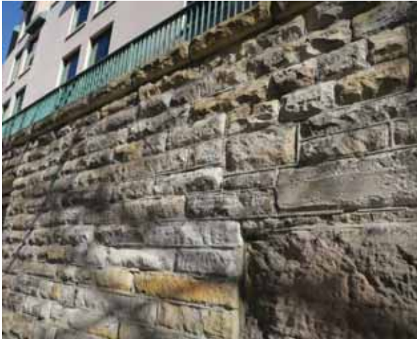
PICTURE 1 – BEDROCK AND RETAINING WALL ON HARRINGTON STREET
