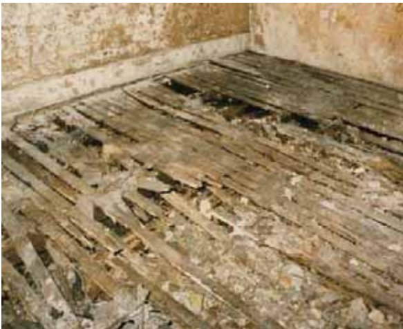
PICTURE 13 – BASEMENT OF NO.72 SOURCE: FUTUREPAST CMP 2006
