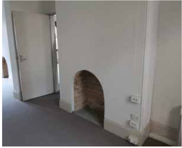
PICTURE 8 – INTERIOR OF BAKERS TERRACE
