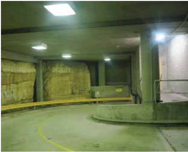
PICTURE 3 – BASEMENT PARKING CUTTING INTO THE BEDROCK
