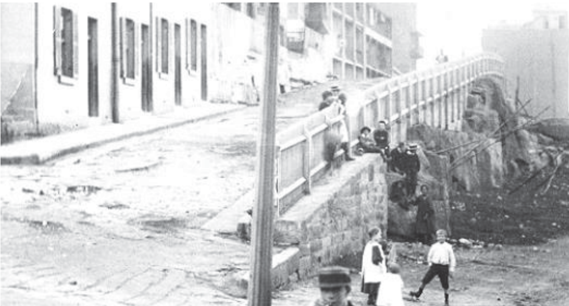
FIGURE 13 – C1901 SHOWING THE CUTTING BACK OF THE ROCK FACE ON HARRINGTON STREET AND PARTIAL CONSTRUCTION OF THE STONE FACING OF THE WALL.
