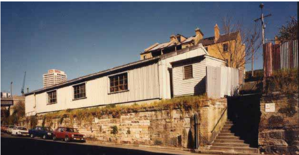
FIGURE 18 – THE STUDY AREA IN 1980 INCLUDING THE STAIRS OF CUMBERLAND PLACE, THE STONE RETAINING WALL AND BAKERS TERRACES IN THE REAR.
