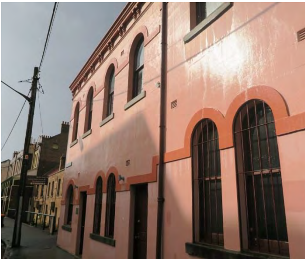
PICTURE 3 – GLOUCESTER STREET FRONTAGE OF BAKER'S TERRACES
