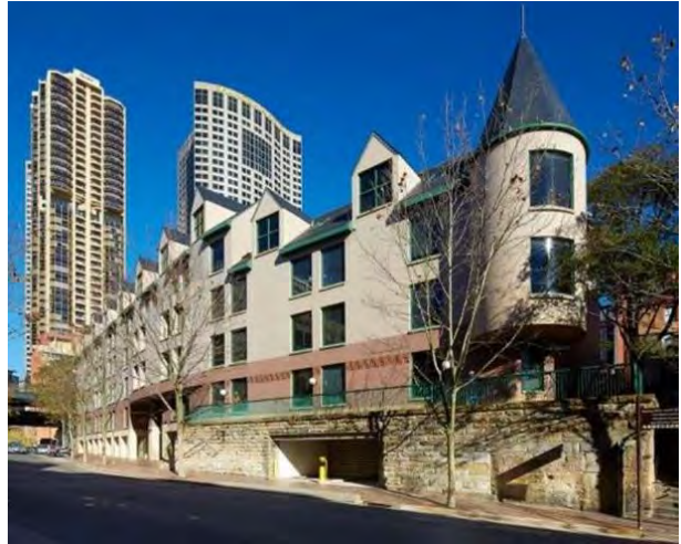
PICTURE 2 – HARRINGTON STREET FACADE (LOOKING SOUTH)
