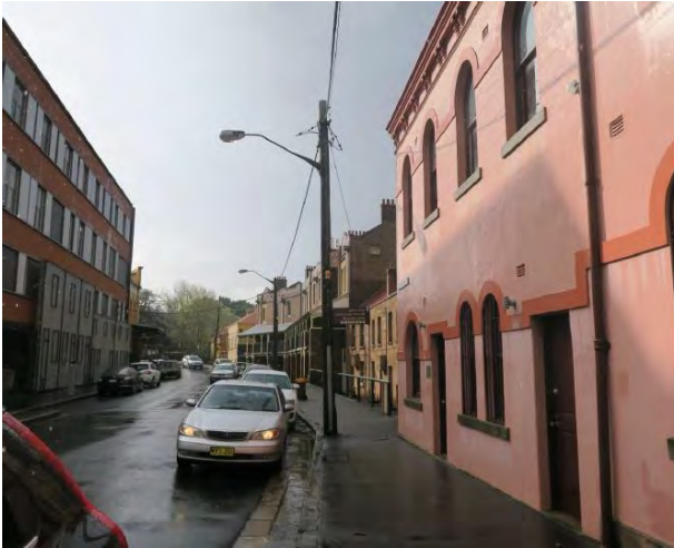
PICTURE 1 – GLOUCESTER STREET FACADE AT BAKER'S TERRACES
