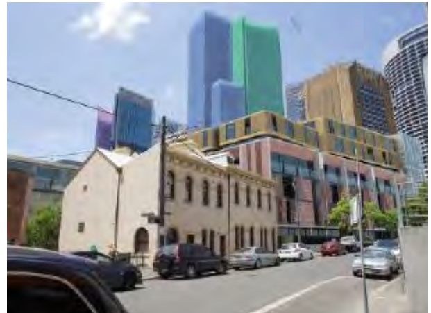
PICTURE 19 – LOOKING NORTH-EAST FROM GLOUCESTER STREET (AFTER)
