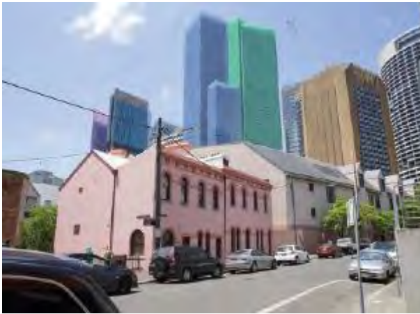
PICTURE 18 – LOOKING NORTH-EAST FROM GLOUCESTER STREET (BEFORE)
