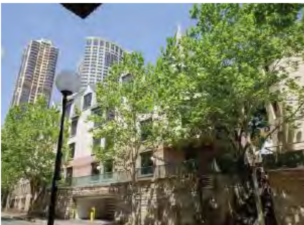
PICTURE 14 – LOOKING SOUTH-WEST ALONG HARRINGTON STREET (BEFORE)
