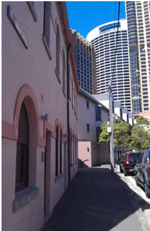
Photo 5 - Baker's Street Terraces facing south
