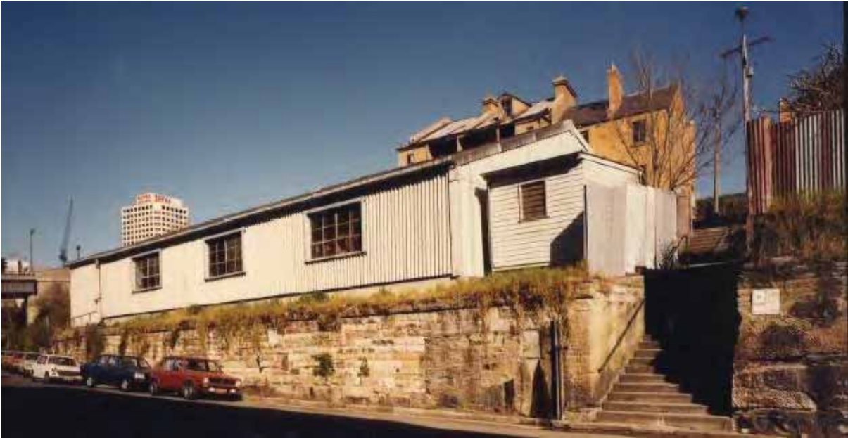
FIGURE 21 – THE STUDY AREA IN 1980 INCLUDING THE STAIRS OF CUMBERLAND PLACE, THE STONE RETAINING WALL AND BAKERS TERRACES IN THE REAR.
