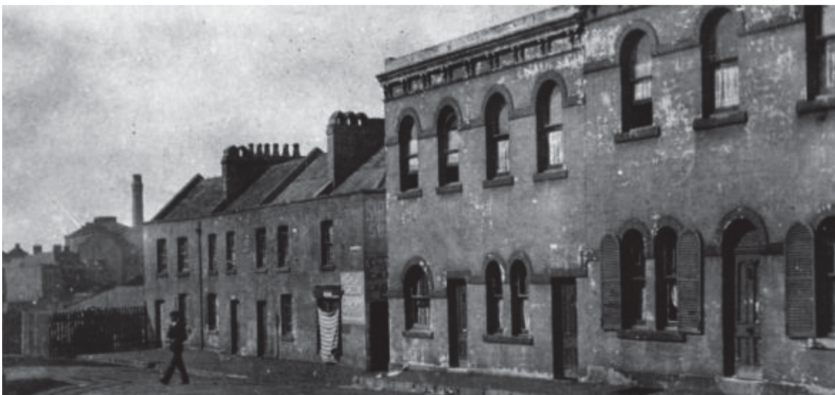
FIGURE 18 – GLOUCESTER STREET SHOWING BAKERS TERRACES, C1910 PRIOR TO THE REALIGNMENT OF GLOUCESTER STREET AND THE RETAINING WALL TO THE FRONT OF SUSANNAH PLACE.
