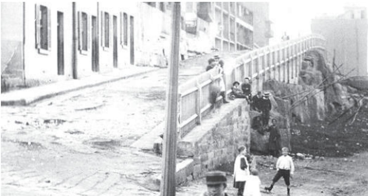
FIGURE 15 – C1901 SHOWING THE CUTTING BACK OF THE ROCK FACE ON HARRINGTON STREET AND PARTIAL CONSTRUCTION OF THE STONE FACING OF THE WALL.
