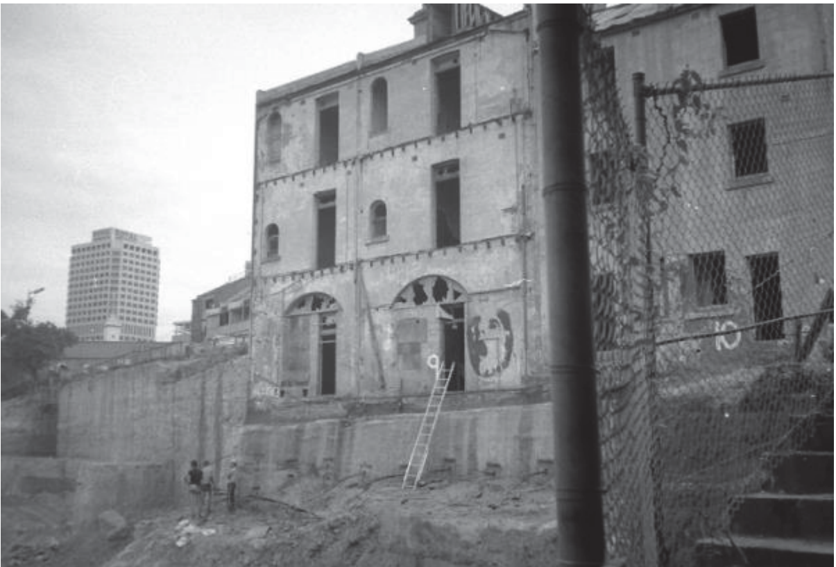
FIGURE 22 – EXCAVATION OF CAMBRIDGE STREET AS PART OF THE LATE 1980S REDEVELOPMENT WORKS FOR THE SUBJECT SITE.
