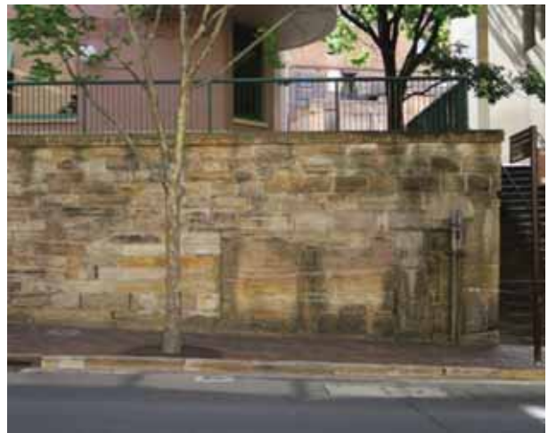
PICTURE 8 – RETAINING WALL AND CUMBERLAND PLACE STAIRS ON THE RIGHT.
