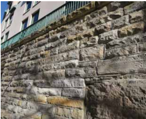
PICTURE 7 – STONE RETAINING WALL TO HARRINGTON STREET.
