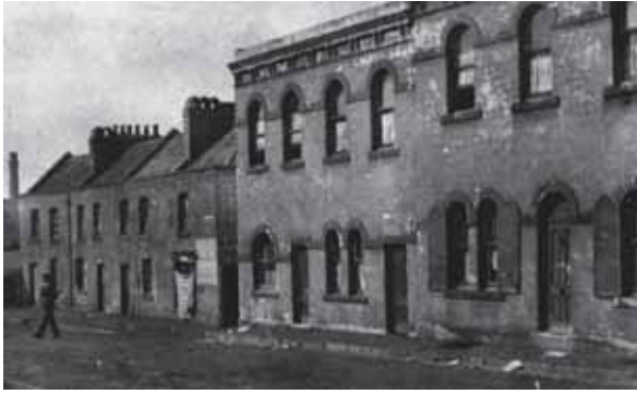
PICTURE 12 – GLOUCESTER STREET SHOWING BAKERS TERRACE. THEY ARE NOTED TO BE VERY DILAPIDATED AND WITH SHUTTERS ON THE LOWER LEVEL SOUTHERN TERRACES. (SOURCE: CMP BAKERS TERRACE, 2007).
