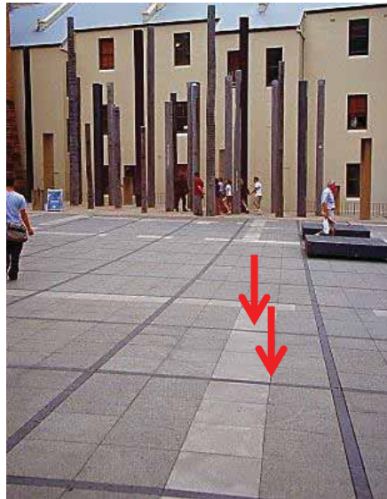
PICTURE 15 – DETAIL OF GROUND INLAYS, WHICH MARK ORIGINAL FOUNDATIONS, EMBEDDED IN LANDSCAPED FORECOURT (SOURCE: HTTPS://WWW.GOOGLE.COM.AU/SEARCH?Q=MUSEUM+OF+SYDNEY+FORECOURT )
