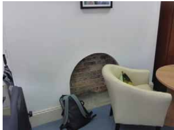
PICTURE 66 – SPACE F1 CHIMNEY DETAIL. (NOVEMBER 2015)
