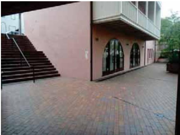
PICTURE 31 – DETAIL OF REAR COURTYARD AND STAIRCASE. (NOVEMBER 2015)
