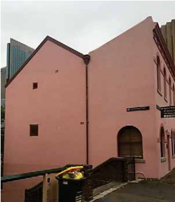
PICTURE 23 – SIDE (NORTH) FAÇADE. (NOVEMBER 2015)
