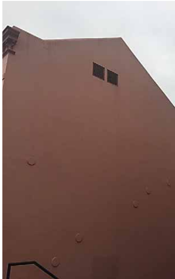
PICTURE 34 – DETAIL OF SIDE (SOUTH) FACADE. (NOVEMBER 2015)
