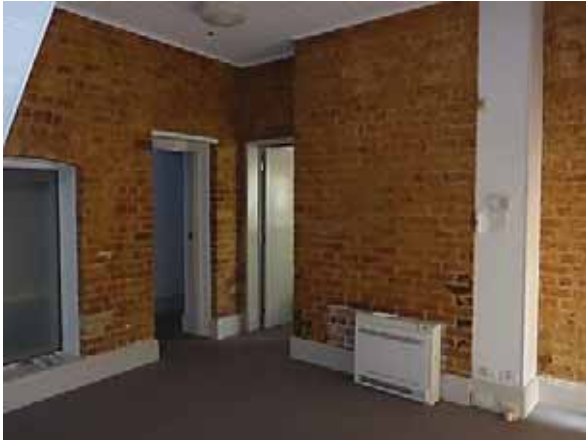
PICTURE 37 – SPACE B1 FACING NORTH WEST (NOVEMBER 2015)
