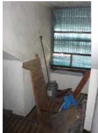
PICTURE 76 – SPACE A1 PLANT ROOM FACING EAST. (NOVEMBER, 2015)
