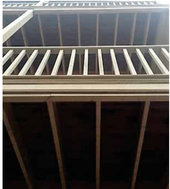
PICTURE 30 – DETAIL OF REAR TIMBER BALCONY. (NOVEMBER 2015)
