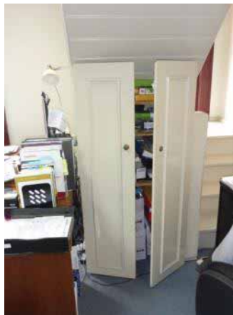
PICTURE 70 – SPACE F7 FACING EAST. (NOVEMBER 2015)
