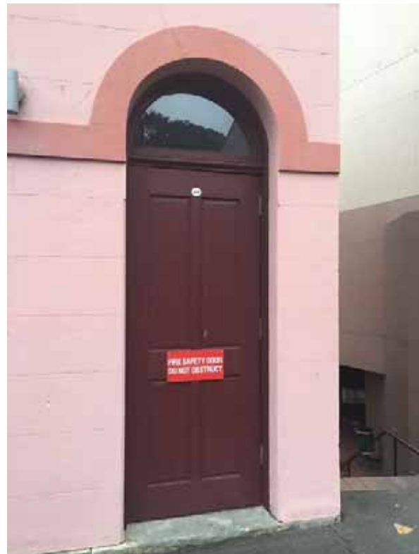
PICTURE 20 – DETAIL OF EXISTING FIRE DOOR ON SOUTHERN END OF NUMBER 72. NOTE ORIGINAL DOOR HIGHLIGHT. (NOVEMBER 2015)
