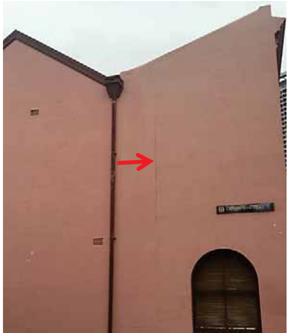
PICTURE 24 – DETAIL OF SIDE (NORTH) FAÇADE WITH RED ARROW SHOWING THE APPROX. LOCATION OF THE LATE 1880S FRONT EXTENSION TO THE NORTHERN TERRACES. (NOVEMBER 2015)
