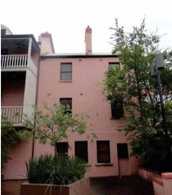
PICTURE 29 – DETAIL OF REAR OF NORTHERN TERRACES. NOTE EXISTING WINDOW ON FAR RIGHT WAS ORIGINALLY A DOOR. (NOVEMBER 2015)
