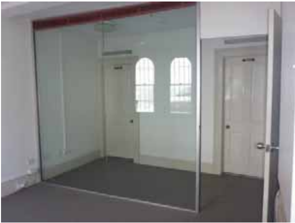
PICTURE 57 – SPACE G4 FACING EAST. NOTE GLASS PARTITION WALL AND PAINTED TIMBER FLUSH DOOR (NOVEMBER 2015)
