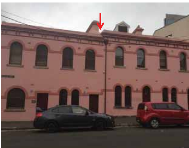
PICTURE 14 – VIEW 5 TO BAKERS TERRACE FROM OPPOSITE SIDE OF GLOUCESTER STREET, URBIS, 2015.
