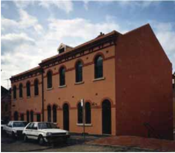
PICTURE 84 – FRONT FAÇADE IMMEDIATELY SHOWING RESTORATION, 1991 (SOURCE: BAKERS TERRACE CMP, 2007)
