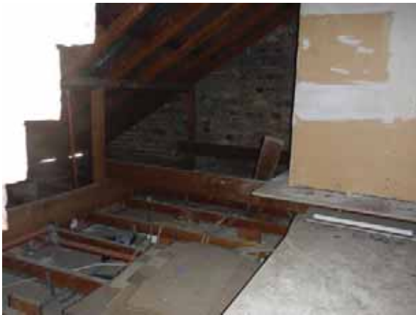
PICTURE 75 – SPACE A1 FACING SOUTH (UNDER ROOF SPACE). (NOVEMBER, 2015)
