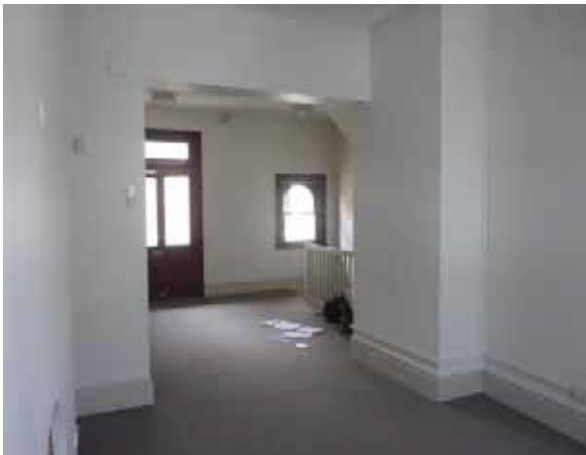
PICTURE 51 – SPACE G2/G9 FACING SOUTH EAST (NOVEMBER 2015)
