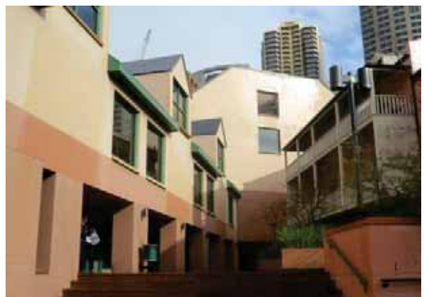
PICTURE 7 – REAR OF BAKERS TERRACE ON RIGHT AND HARRINGTON COURT ON LEFT.
