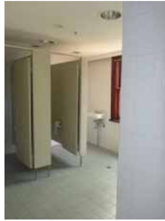
PICTURE 62 – SPACE G6 FACING NORTH EAST. (NOVEMBER 2015)
