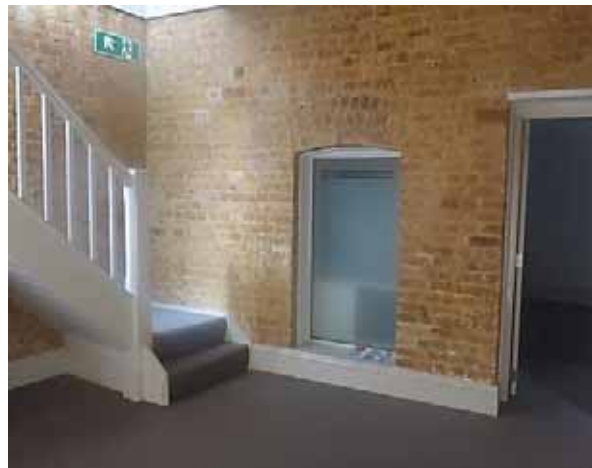
PICTURE 36 – SPACE B1, FACING SOUTH WEST (NOVEMBER 2015)
