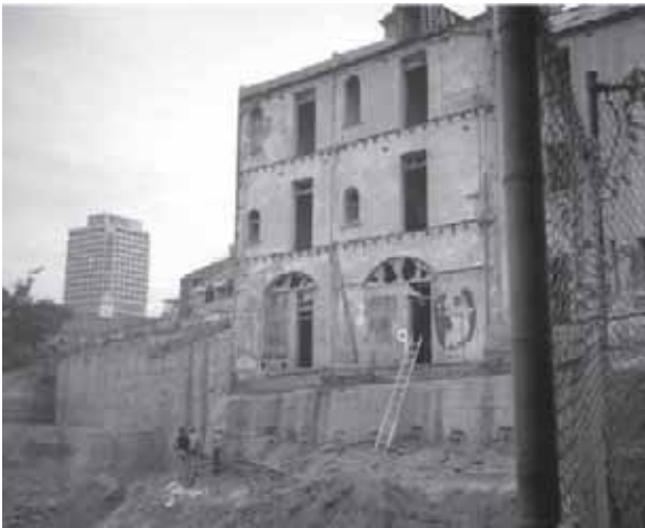
PICTURE 80 – REAR FAÇADE SHOWING EXTENSIVE DEMOLITION AND EXCAVATION UNDERTAKEN AT REAR, C1988 (SOURCE: BAKERS TERRACE CMP, 2007)
