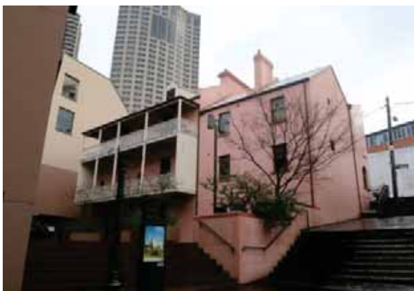
PICTURE 6 – REAR ELEVATION OF BAKERS TERRACE FROM CUMBERLAND PLACE AND STEPS.
