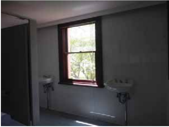
PICTURE 61 – SPACE G6 FACING NORTH EAST. (NOVEMBER 2015)
