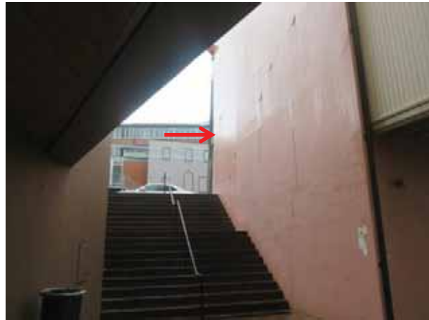
PICTURE 17 –VIEW 8 TO THE SOUTHERN FAÇADE OF BAKERS TERRACE FROM HARRINGTON COURT DEVELOPMENT, URBIS, 2015.
