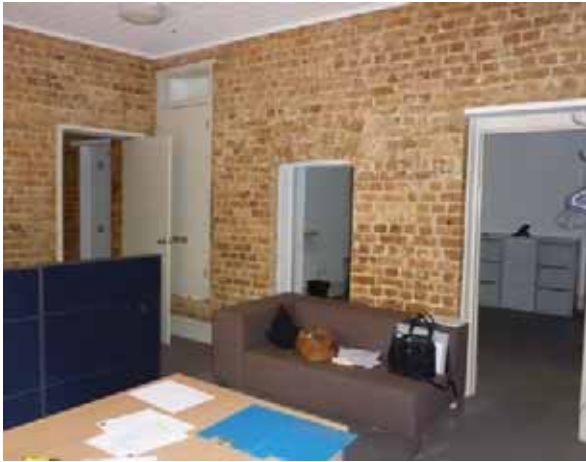
PICTURE 39 – SPACE B2 FACING SOUTH WEST (NOVEMBER 2015)
