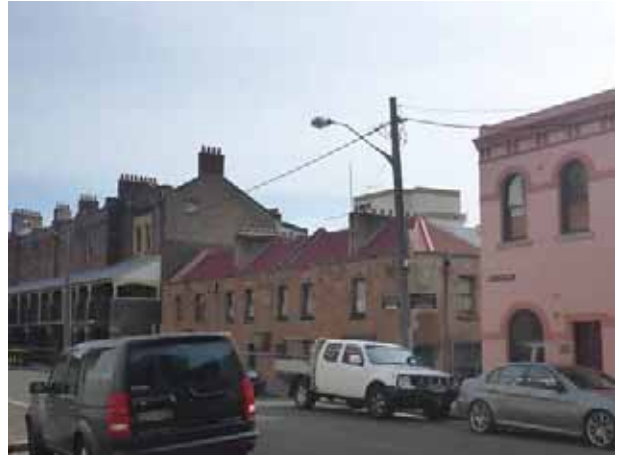
PICTURE 2 – GLOUCESTER STREET STREETScape, SHOWING SUSANNAH PLACE TO THE NORTH OF BAKERS TERRACE.
