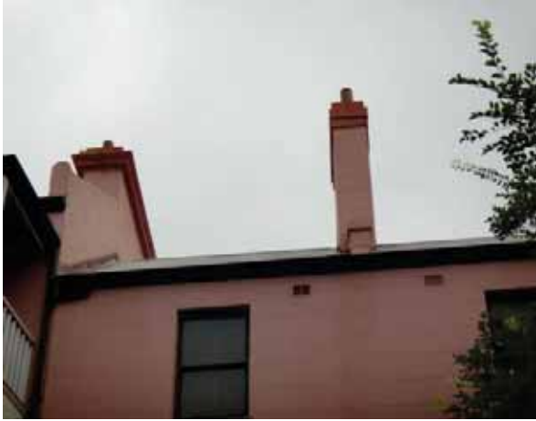
PICTURE 27 – DETAIL OF REAR ROOF AND CHIMNEY. (NOVEMBER 2015)
