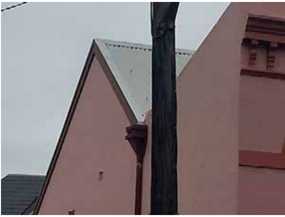
PICTURE 21 – DETAIL OF EXISTING PAINTED METAL ROOF SHEETING. (NOVEMBER 2015)
