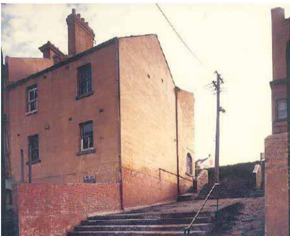
PICTURE 82 – REAR OF THE BUILDINGS DURING THE C1988 RENOVATIONS (SOURCE: BAKERS TERRACE CMP, 2007)
