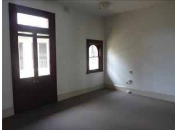
PICTURE 56 – SPACE G8 FACING SOUTH EAST. (NOVEMBER 2015)
