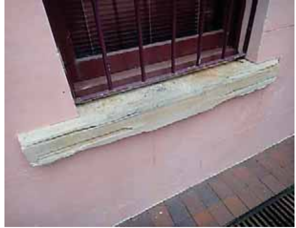
PICTURE 28 – DETAIL OF ORIGINAL REAR SANDSTONE WINDOW SILL. (NOVEMBER 2015)
