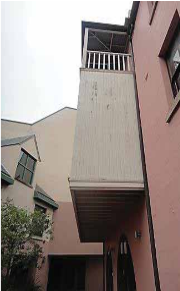
PICTURE 33 – DETAIL OF REAR BALCONY. (NOVEMBER 2015)
