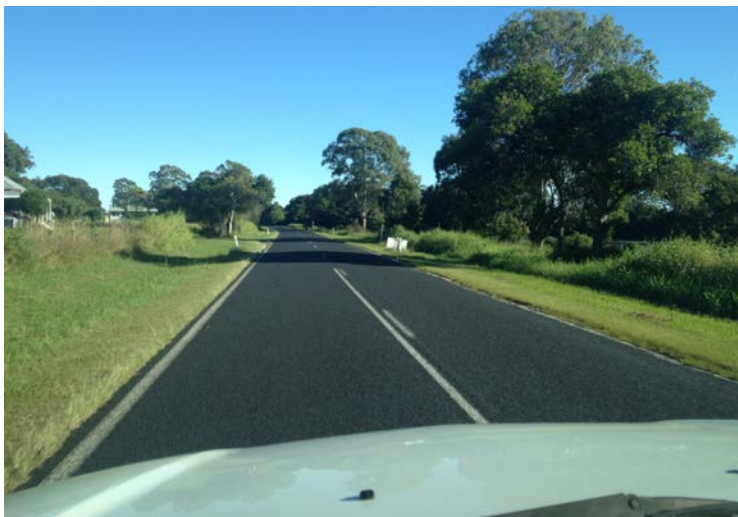
Figure 2-7: Coraki Woodburn Road looking north-west
