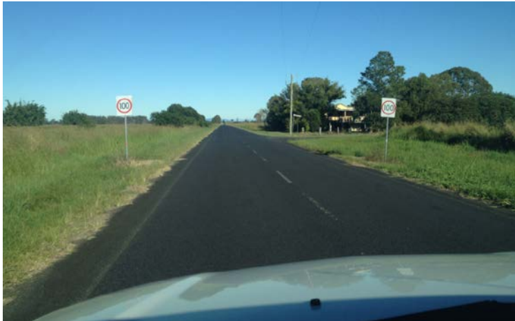
Figure 2-4: Lagoon Road looking west
