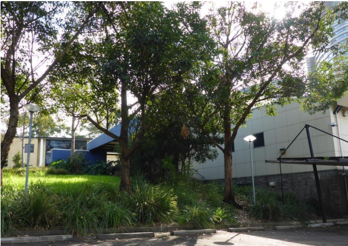
FIGURE 6 – REAR OF THE BUILDING STEPPING DOWN THE SITE
