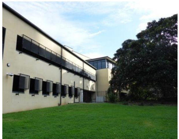
PICTURE 6 – NORTH EASTERN FAÇADE
