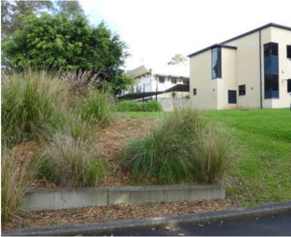
PICTURE 7 – VIEW FROM AUSTRALIA AVE SHOWING CUTTING BACK OF THE LANDFORM FOR THE ROAD AND FOOTPATH
