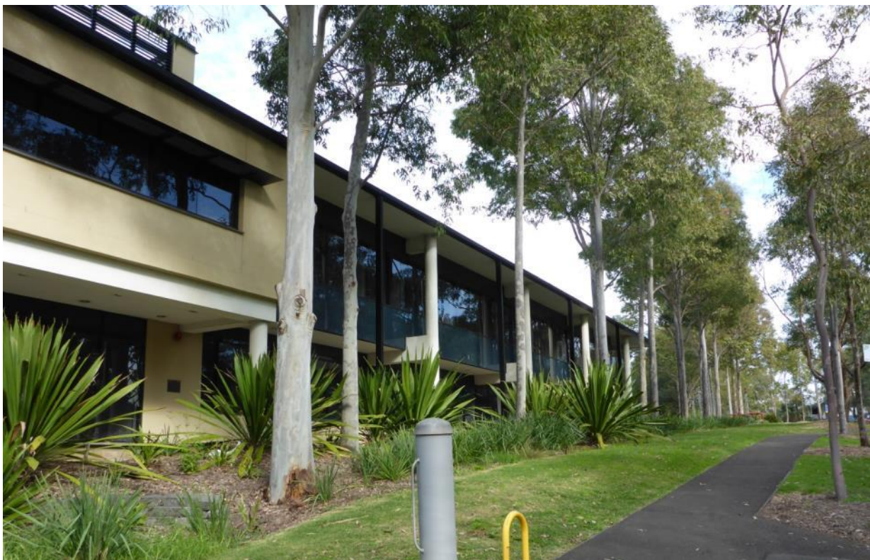
FIGURE 3 – FRONT FAÇADE OF CURRENT BUILDING ON THE SITE
