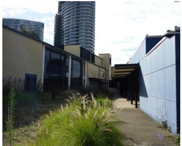
PICTURE 4 – COURT YARD BETWEEN THE TWO BUILDINGS
