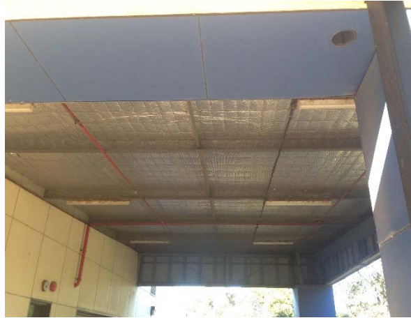
Photograph 8: Roof of the loading dock on the western side of Building one
