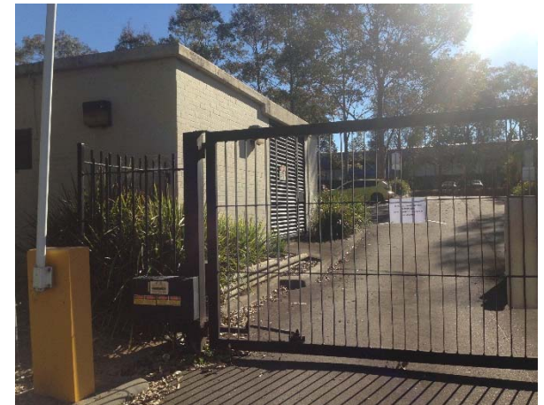
Photograph 12: Southern side of Building three and automatic gate.
