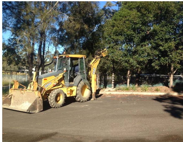
Photograph 17: Location of BH02 in the south western corner
