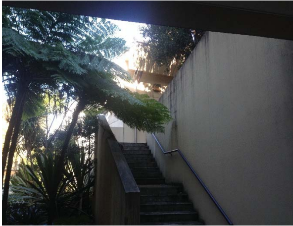
Photograph 13: Concrete stairs connecting the upper Building on level and the lower Building two level
