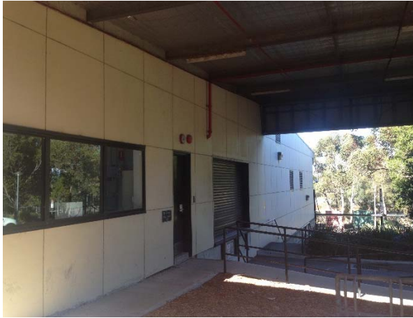
Photograph 7: Western side of Building two showing the loading dock
