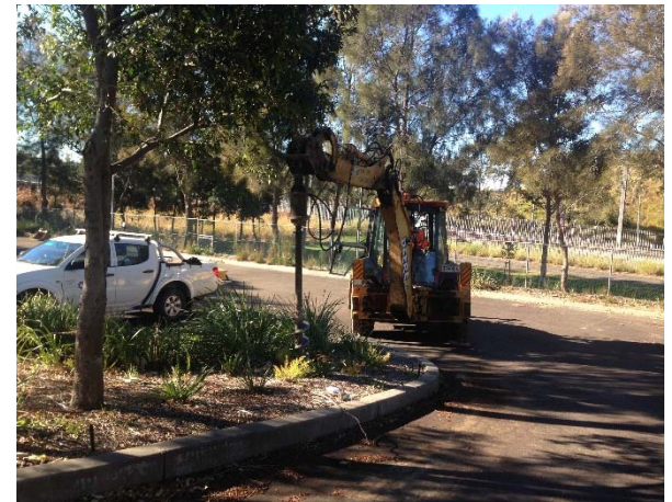
Photograph 18: Location of BH03 in the garden bed in the south western portion of the car park
