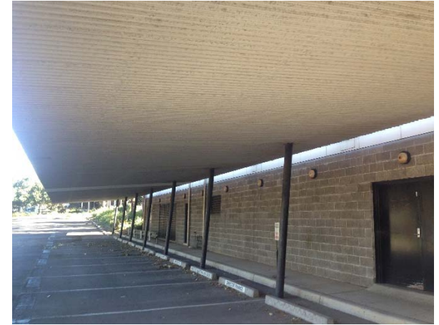
Photograph 9: Car park cover on the southern side of Building two
