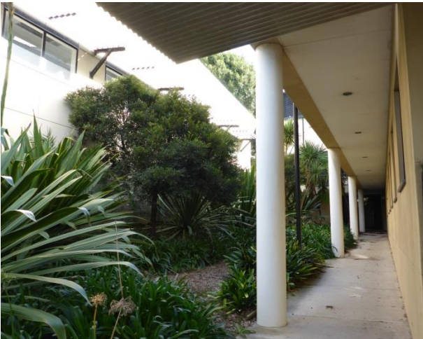
PICTURE 7 – COURT YARD BETWEEN TWO SECTIONS OF THE BUILDING
