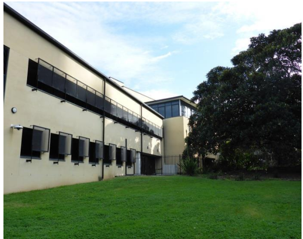
PICTURE 8 – NORTH EASTERN FAÇADE
