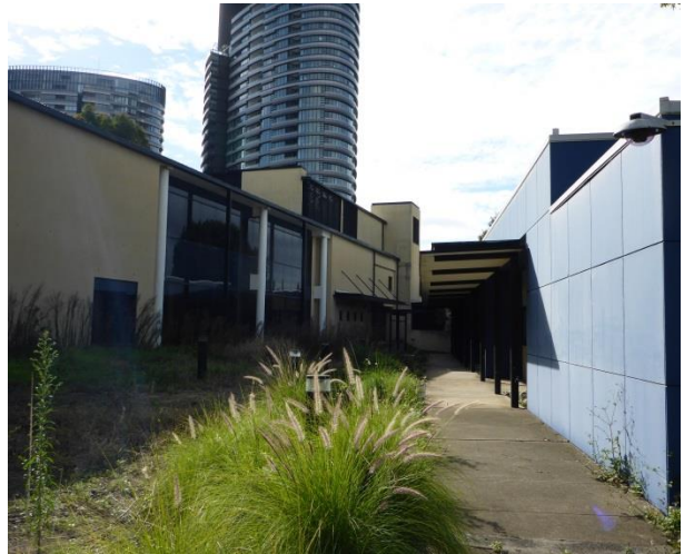
PICTURE 6 – COURT YARD BETWEEN THE TWO BUILDINGS, SHOWING MULTI-STOREY DEVELOPMENT TO THE EAST
