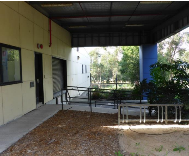
PICTURE 5 – REAR FACADE AND CAR PARK
