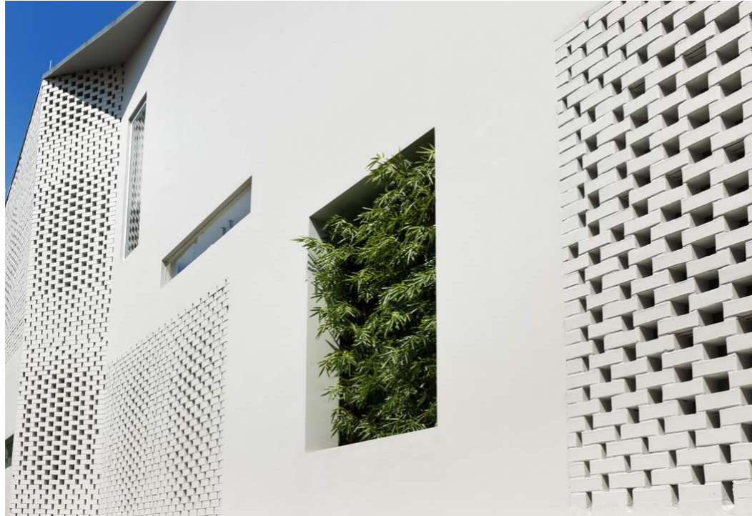
LORONG M TELOK KURAU HOUSE BY A D LAB Pty Ltd 'Hit and Miss' brickwork
