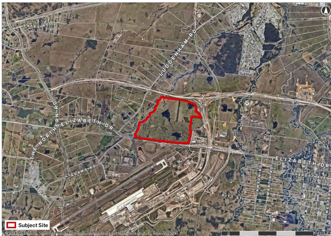
Figure 1: Location of the subject site and regional context (Source: Nearmap and Urbis)
