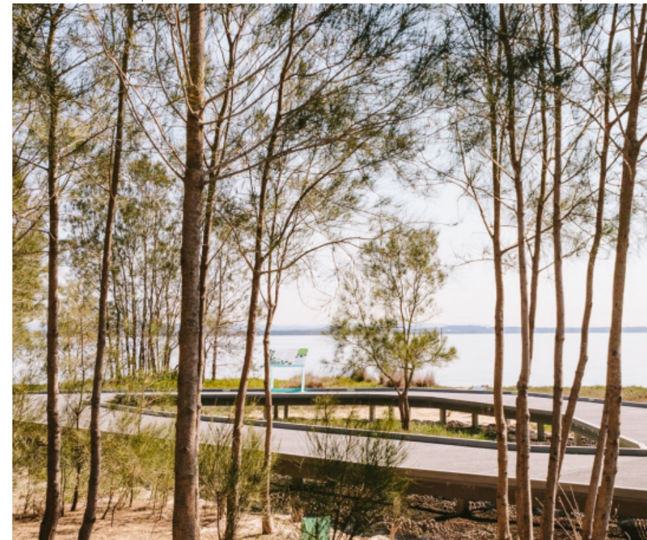
Saltwater Creek Boardwalk | NSW Government
