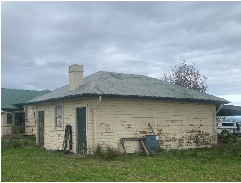
Print 19 Auxiliary building View of the auxiliary building from the east.
