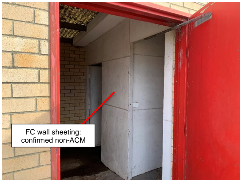
Print 29 Toilet block Internal view of the toilet block. Sample of wall sheeting (SY-TOILETBLOCK) collected and confirmed non-ACM.
