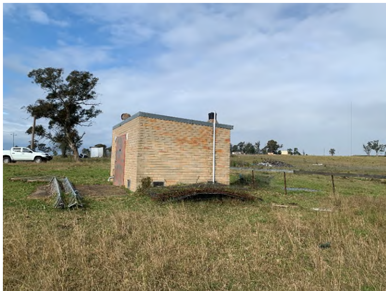
Print 28 Toilet block View of the toilet block from the north.
