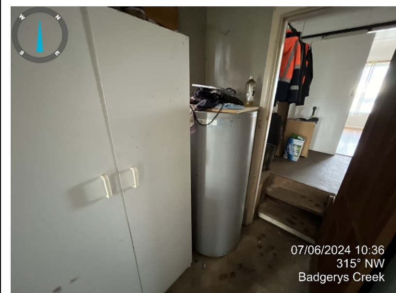
Print 62 Tenanted house Laundry area looking back to store room
