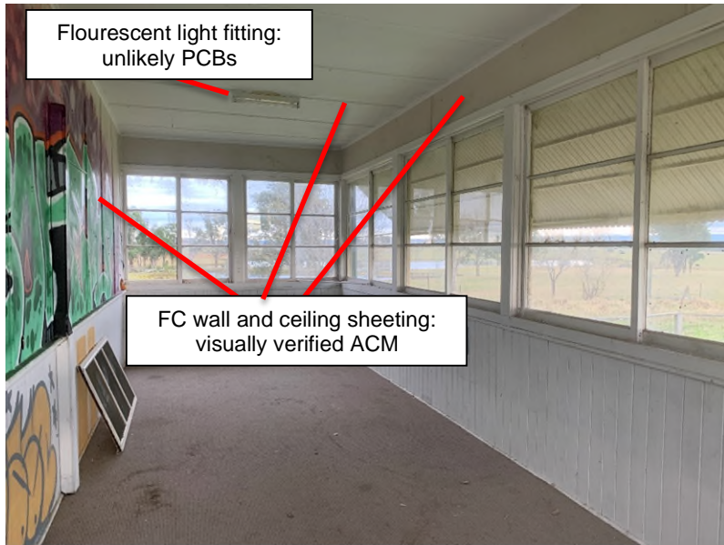
Print 16 Unoccupied house Sunroom at the northwest of the house.
