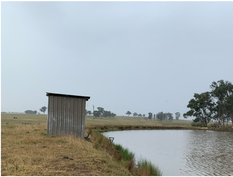
Print 75 Pump house 2 View of pump house 2 from the west.
