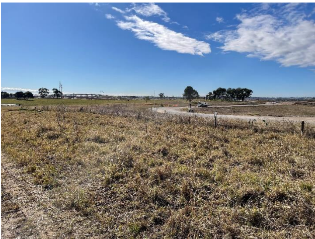
Picture 3 M12 motorway construction
