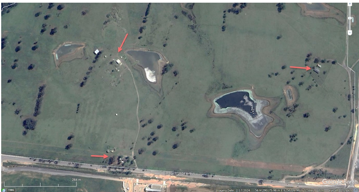
Figure 23. 2024 Air photo showing DAH buildings mostly demolished
