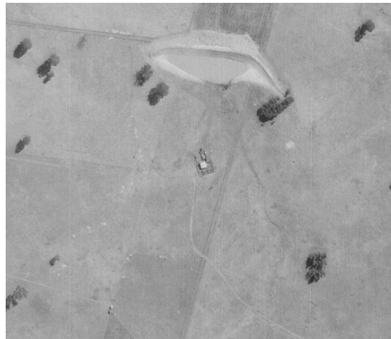
Figure 9. 1955 aerial showing new dam construction
