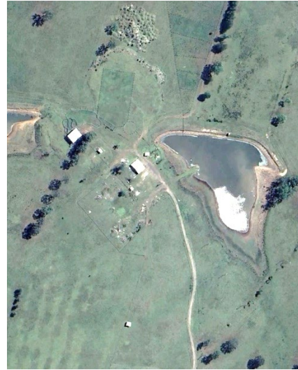
Figure 15. 2024 aerial DAH building complex dilapidation
