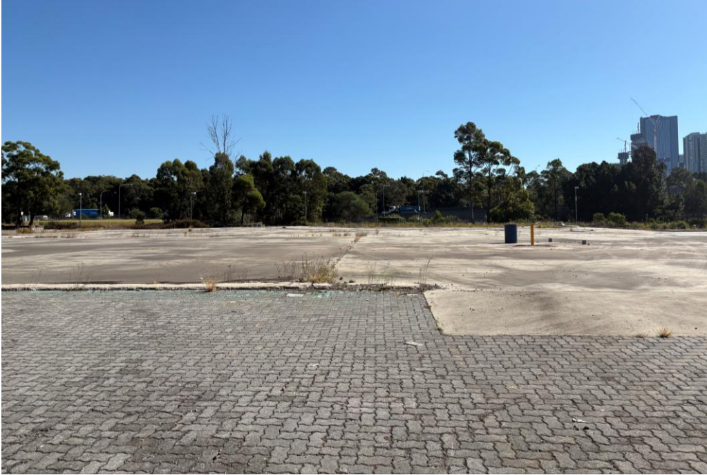
Photo 1: View south to north across cleared hardstand and paving
