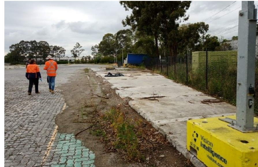
Figure 14: View southeast of the former ancillary building foundation
