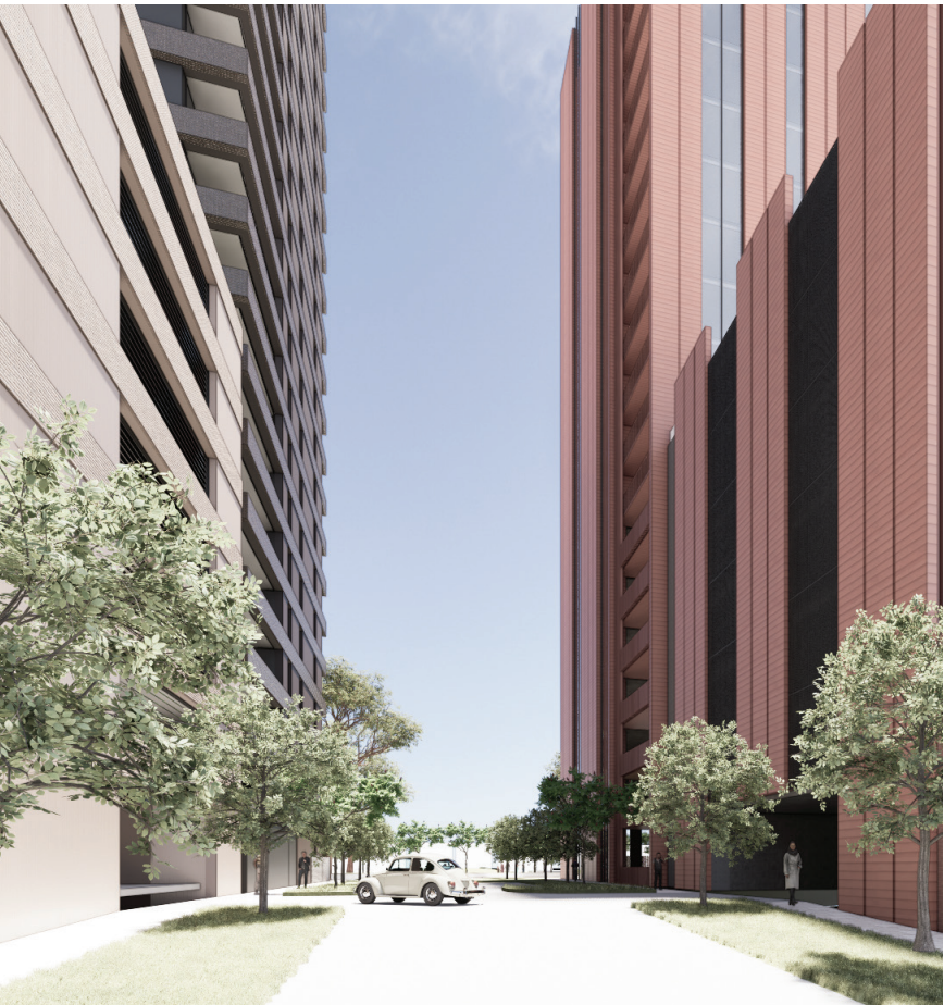
Building 5 - Internal Street and access to carparks
