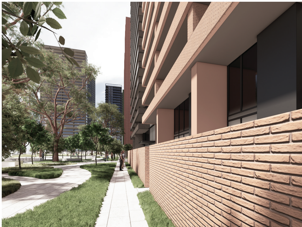
Building 6 - Internal Street frontage.
