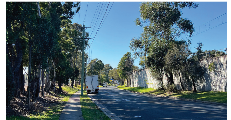
South Edge - Crescent Street
