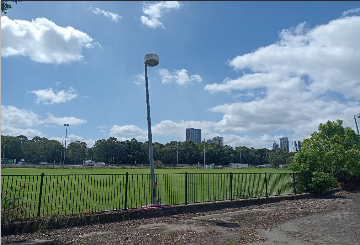
Photo 7: Northern street lights, along northern boundary fence, internal components (e.g. capacitors, ballasts), PCB (suspected).
