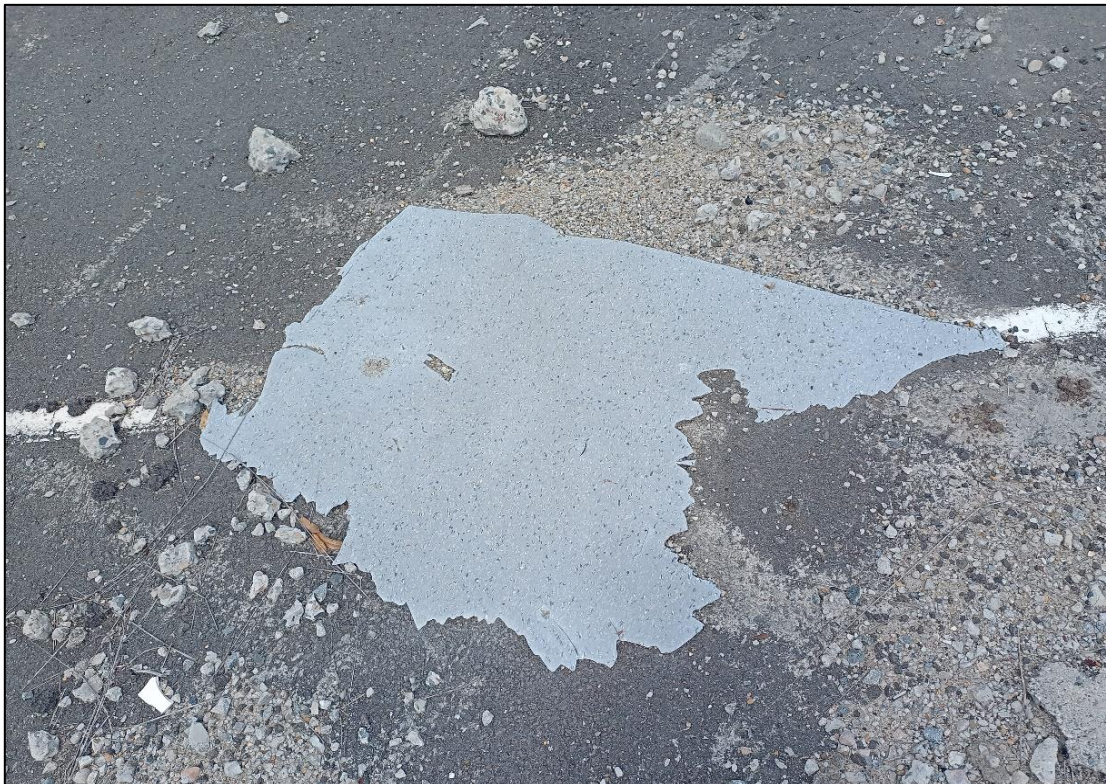
Photo 4: Floor Linoleum, building footprint / north-eastern area, surface, linoleum 1, no asbestos detected by analysis.
