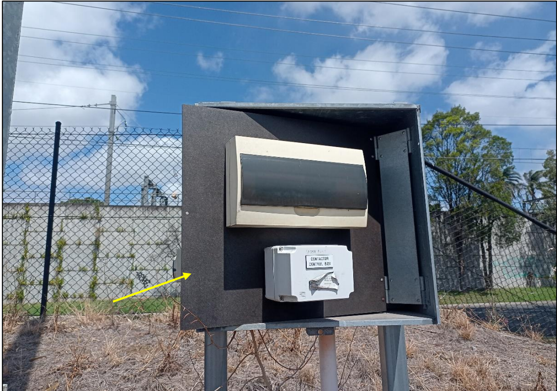
Photo 1: Electrical panel electrical backing board, fibrous cement, asbestos detected by analysis.
