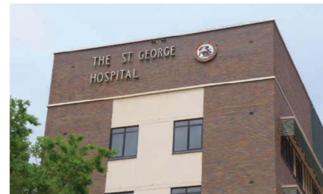
Detail of Ward Block parapet
