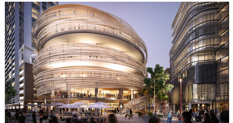
Figure 3.1.2_Timber ribbons are composed in organic patterns which express the dynamic nature of the building.
