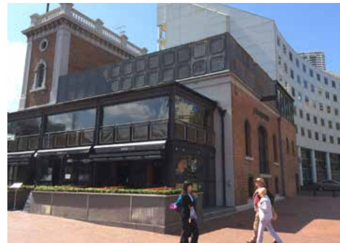
Figure 4.1.7_Photos of Local Context (Pump House)
