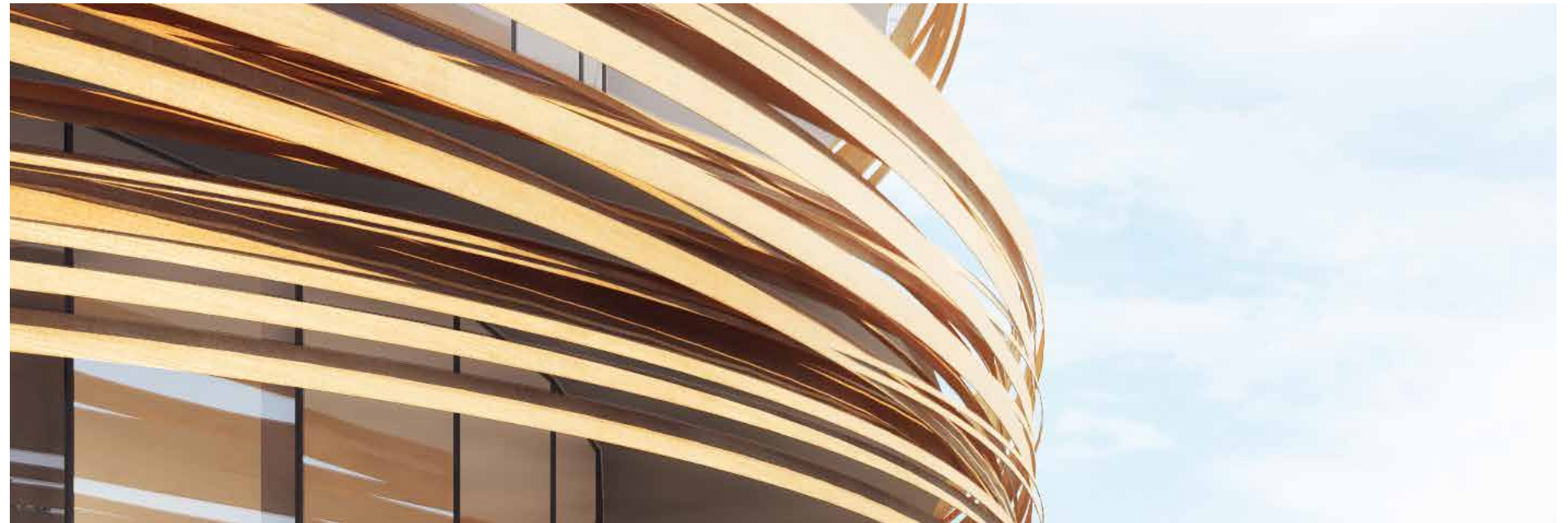
Figure 7.4.1_Close Up View of the Facade
