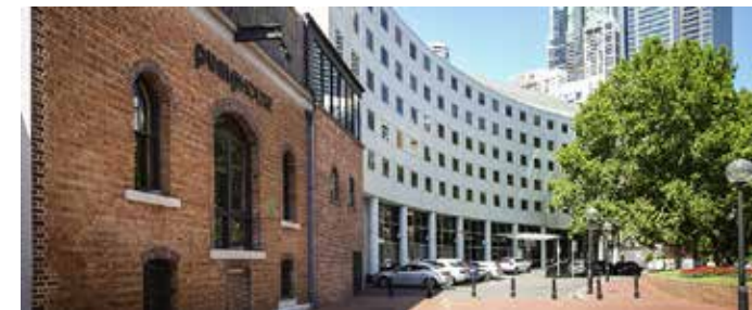
Figure 4.1.6_View of Pump House, Novotel Hotel and Little Pier Street
