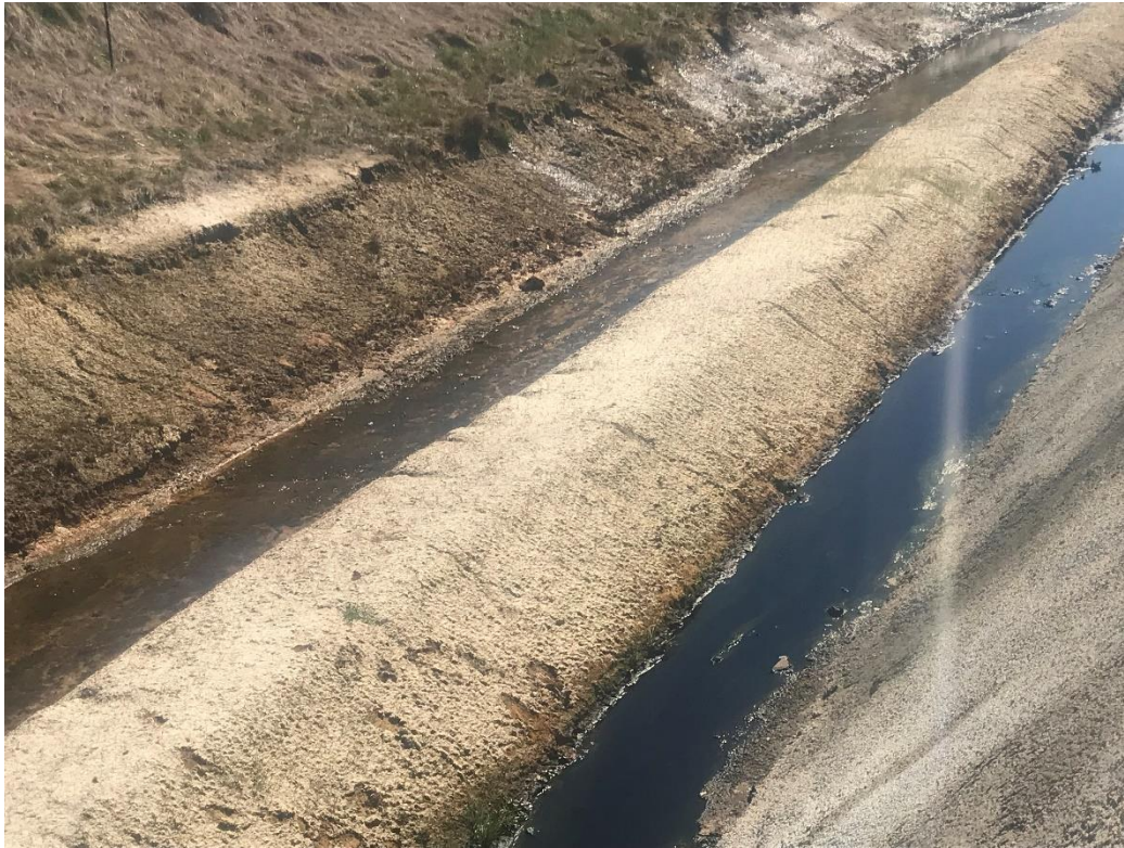
Image 3 – Perimeter swale to the basin and overflow swale to the discharge point.
