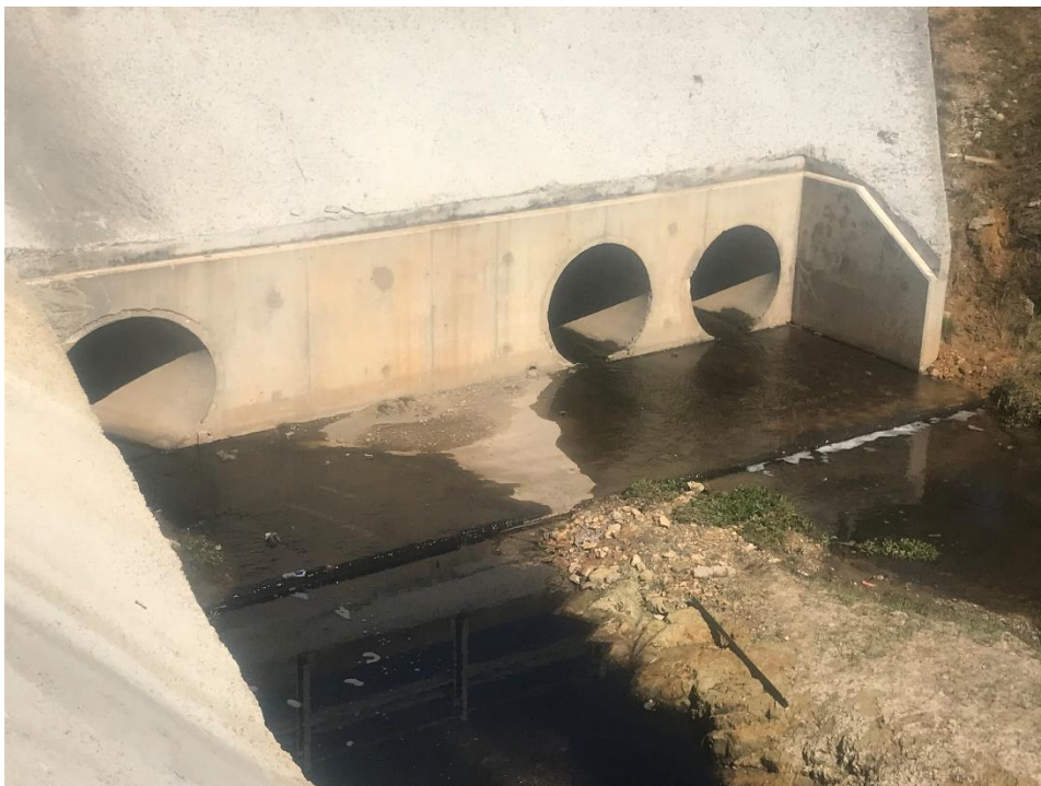
Image 2 – Pipe culvert outlet (showing the internal flow (left) and inflows from adjacent site
