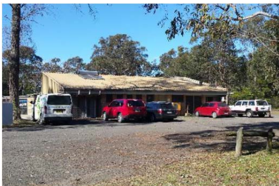
Photo 4.1 Main animal shelter building and car park
