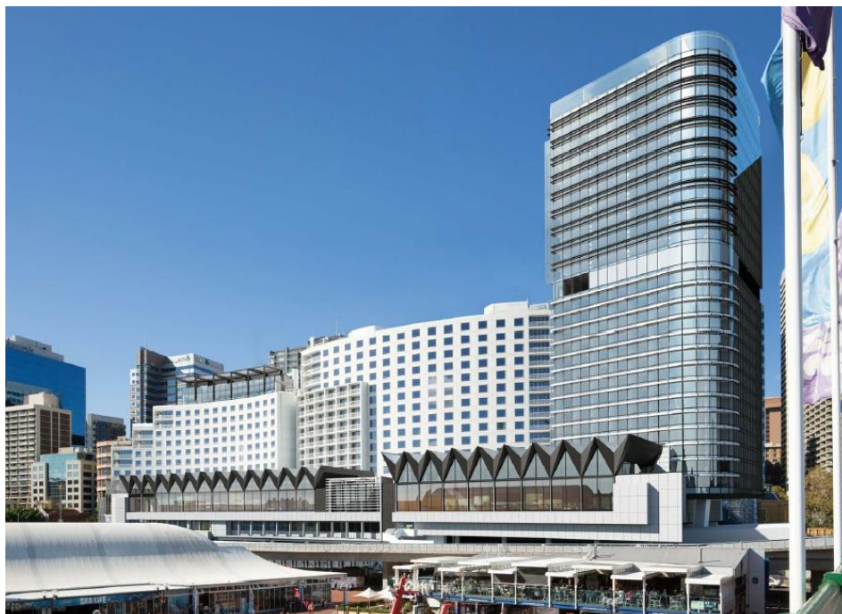
Figure 6 – Photo montage of the proposal, incorporating the approved and proposed elements of SSD 4972 Source: Cox Richardson
