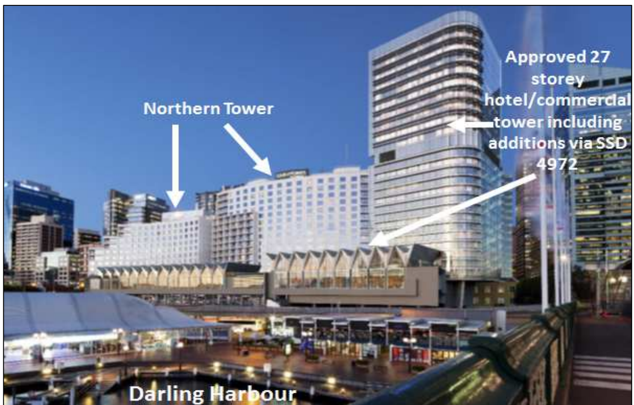
Figure 3: Photomontage of the Sheraton Hotel including the approved commercial/hotel tower and additions at the podium facing Darling Harbour (currently under construction) as viewed from Pyrmont Bridge
