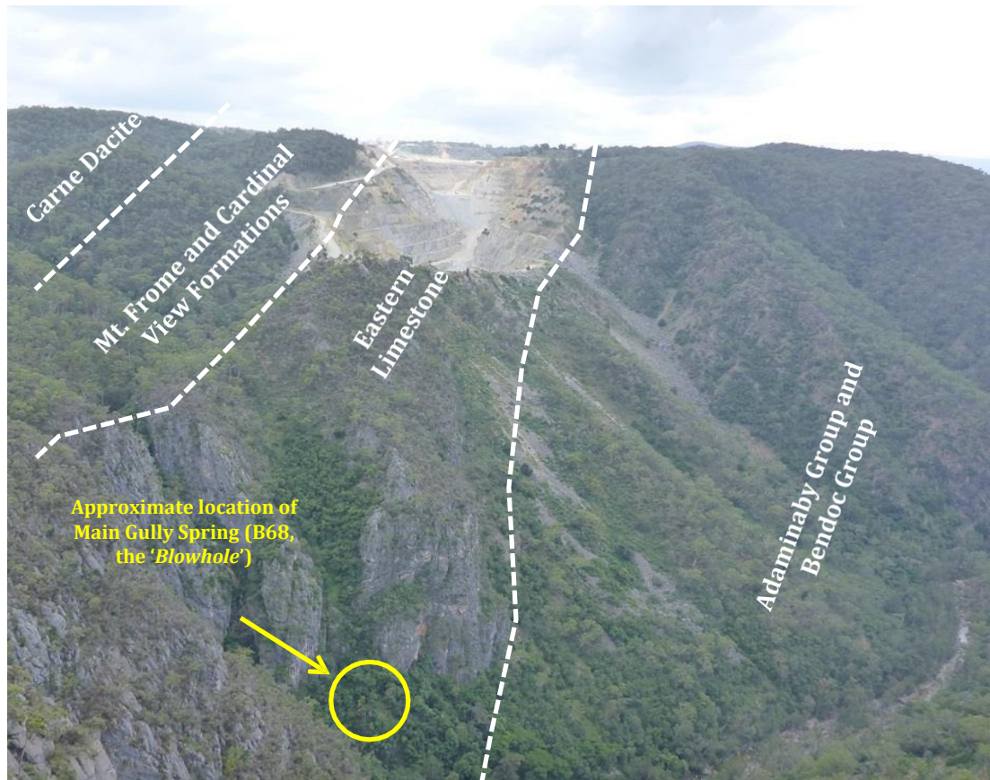
Figure 3.1 View North from Bungonia Gorge lookout - generalised geology and approximate geological boundaries
