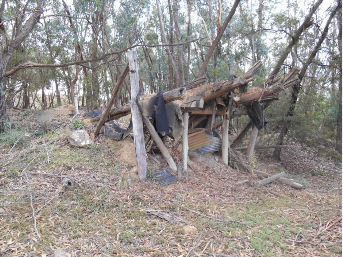
Plate 3.37 MS11 loading ramp (DSCN1067). View north-west.
