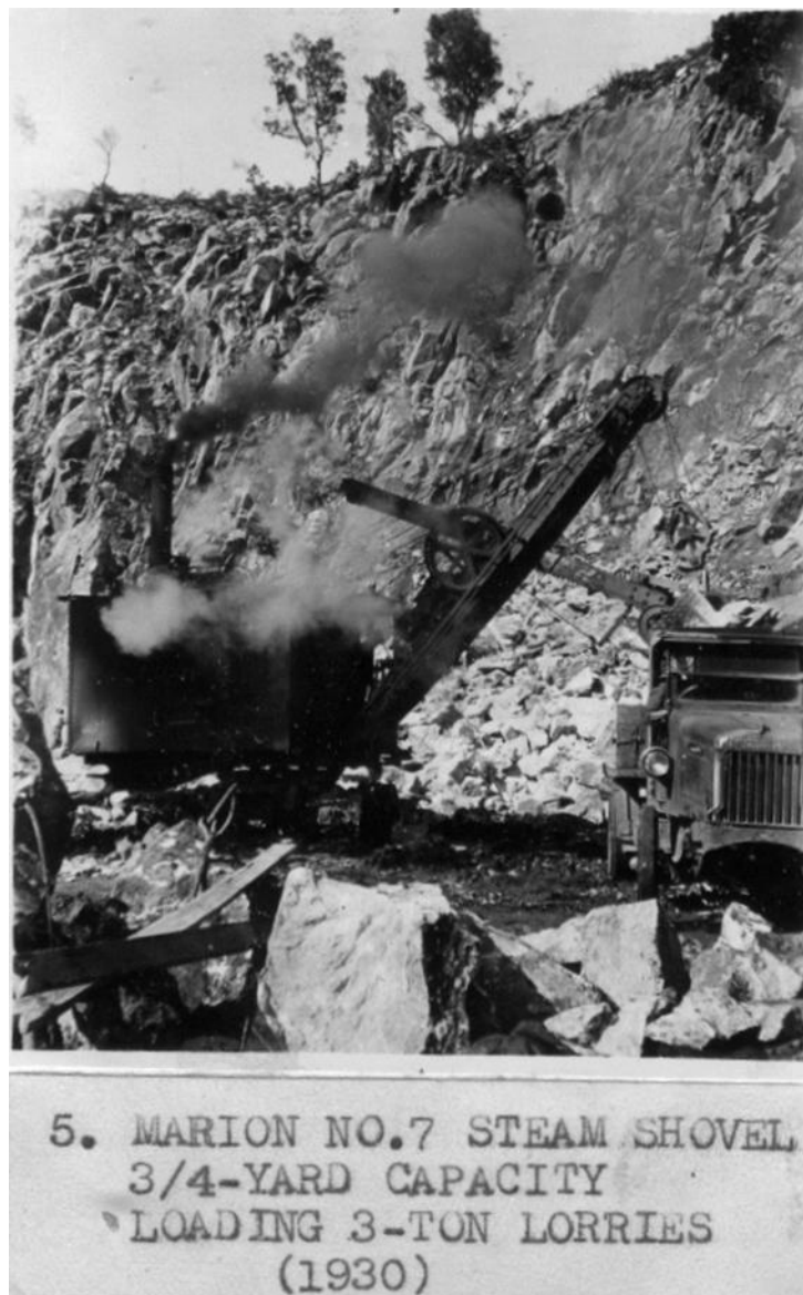
Plate 2.14 An example of the steam shovel and lorries used in the mine in the 1930s (Boral Cement Limited 2015).
