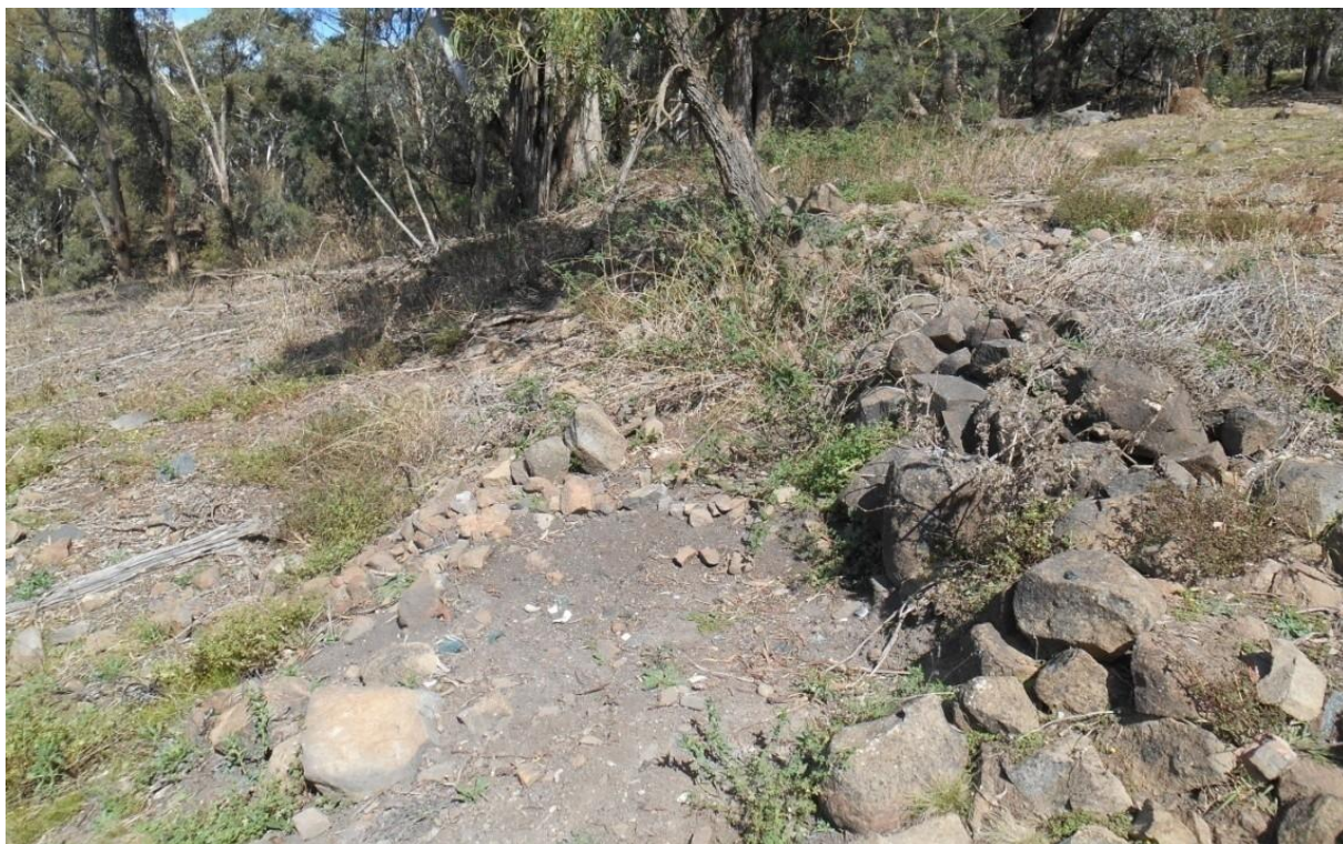
Plate 3.30 MS14 showing close up of possible retaining wall and dump of glass and ceramic (DSM1261). View south.
