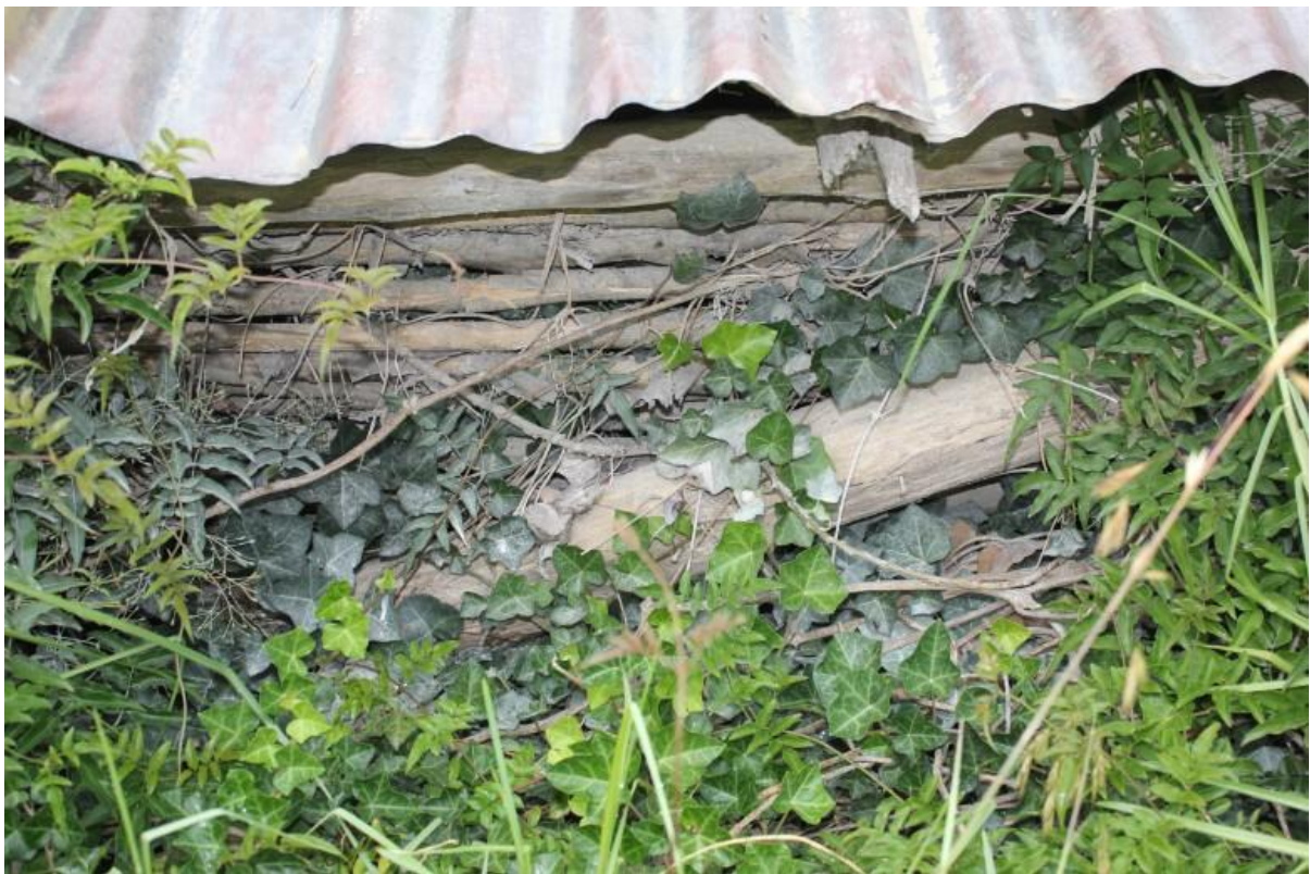
Plate 3.20 MS02 detail of the dilapidated building (above) showing possible wattle and daub construction (IMG_8951).
