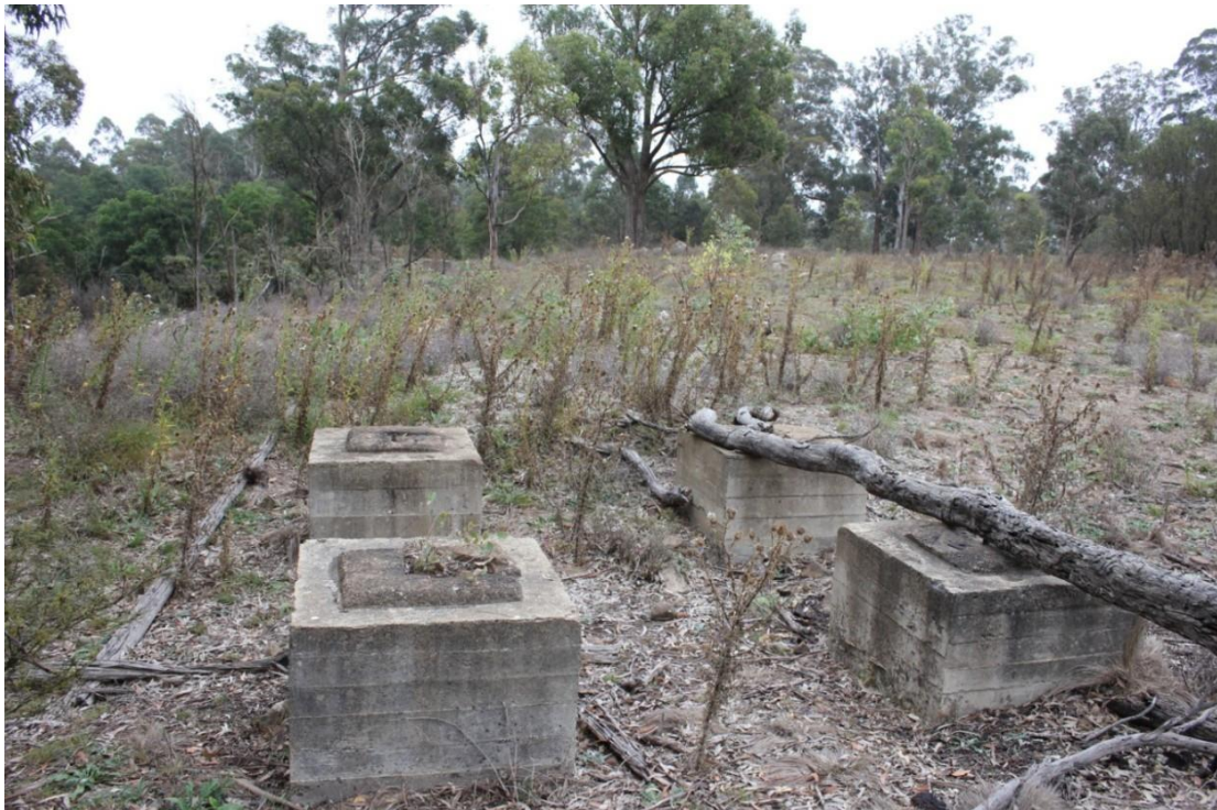
Plate 3.7 Example of groups of concrete plinths (IMG_8990).
