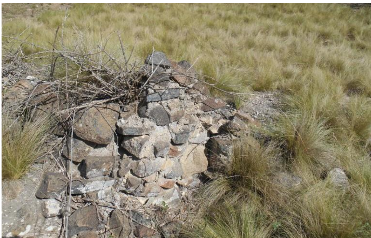
Plate 3.31 MS14 close-up of what appears to be a chimney (DSCN1248). View south-west.
