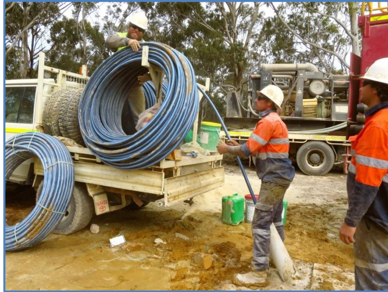
Figure 41 Installing piezometer in hole ML27
