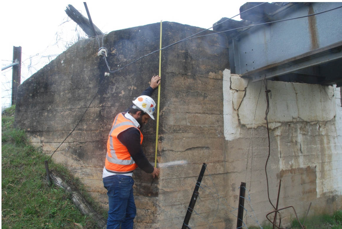
Photo 2: Rail bridge – South abutment – White paint mark is RL597.0 m, measured height to top of concrete is 1.7 m
