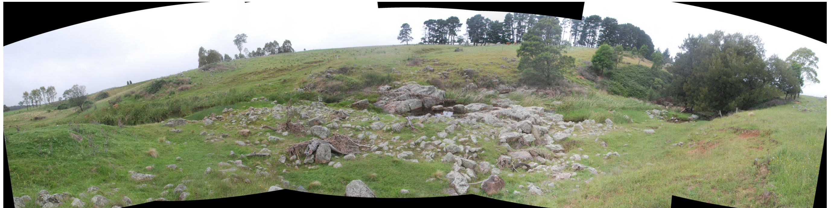
Photo 11: Marulan creek – Dam location C panorama– Trees can be seen at right of photos. Dam Location C centre line approximately at centre of photo. Note rocky foundation
