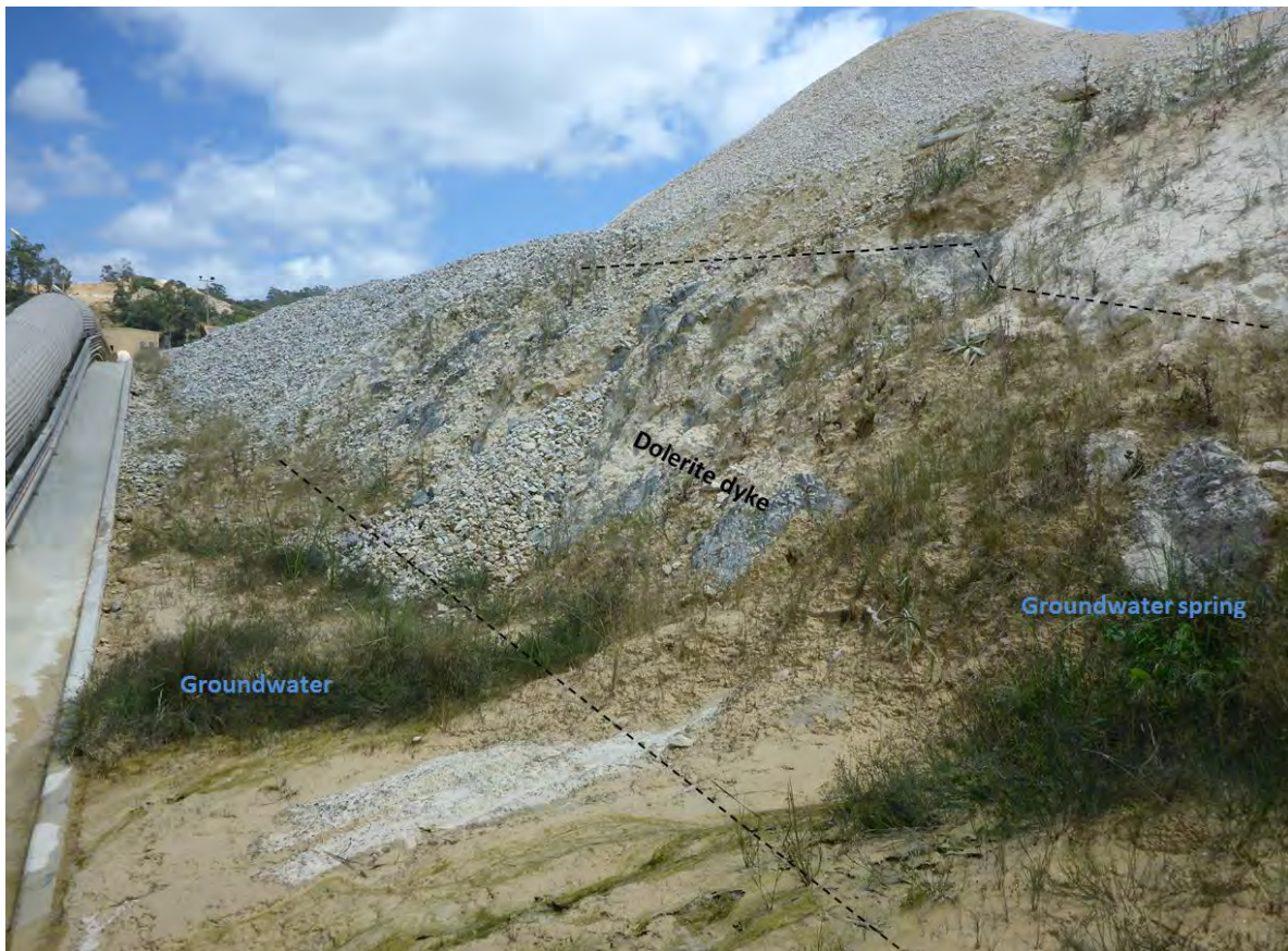
Figure 7-13 North pit dolerite dyke and groundwater spring
