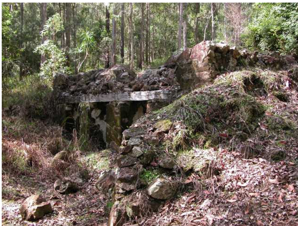
Plate 4.2 Pipers Creek lime kilns showing front wall made of stone (OEH 2015).
