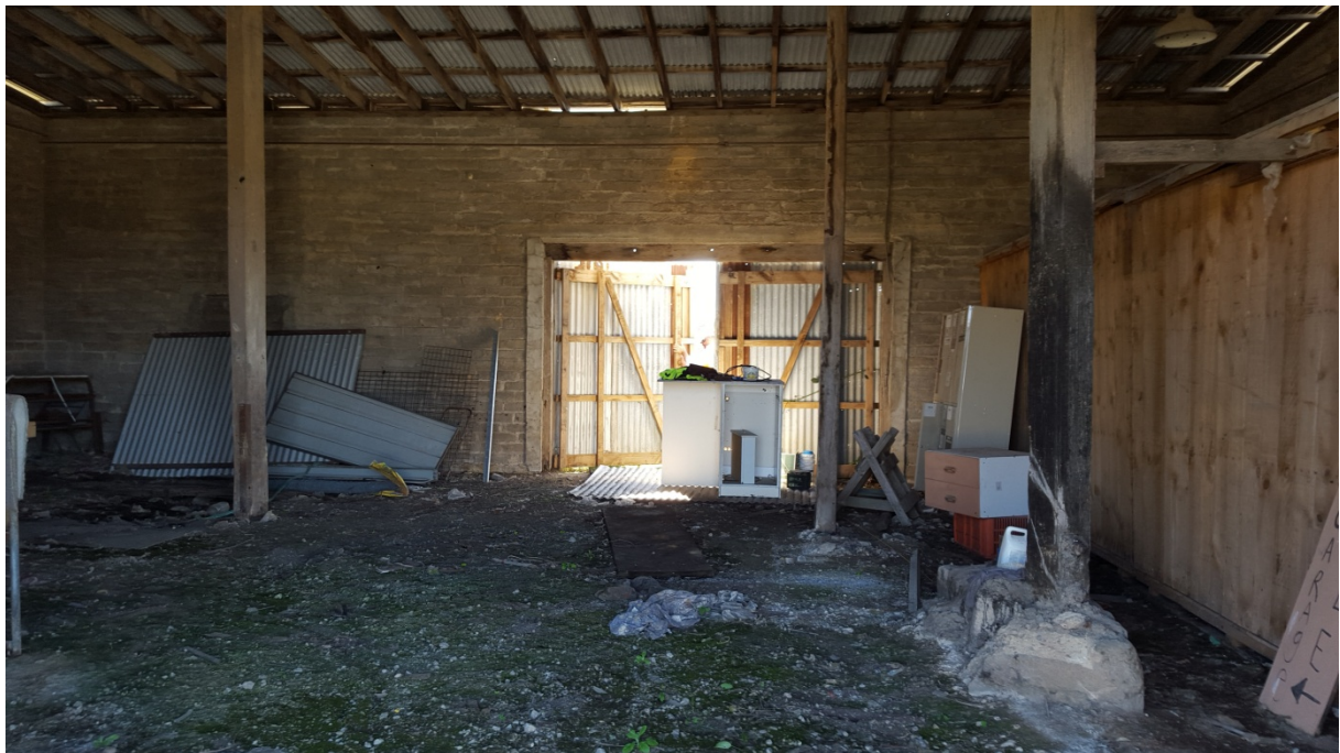
Plate 3.13 Interior of control room showing wooden beams for piles and roof, concrete foundations and dirt floor (20151006_144957).
