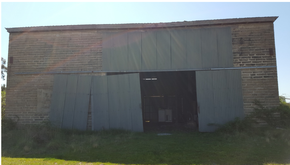
Plate 3.11 Front of the control room (MS04_11), facing west, showing the corrugated iron rolling doors which would have opened to let out heat (at the base) and for the rope to rotate (top) (20151006_144642).
