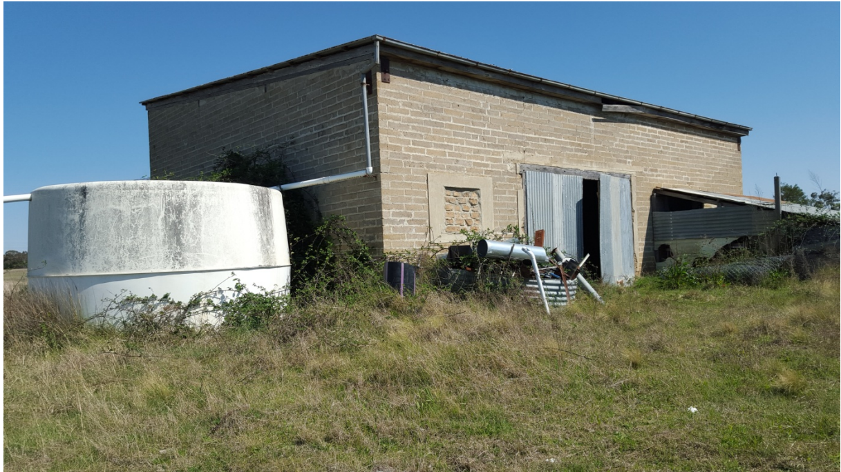
Plate 3.12 Rear of the control room showing corrugated iron engine housing, doors, bricked in openings and a water tank (20151006_145129).
