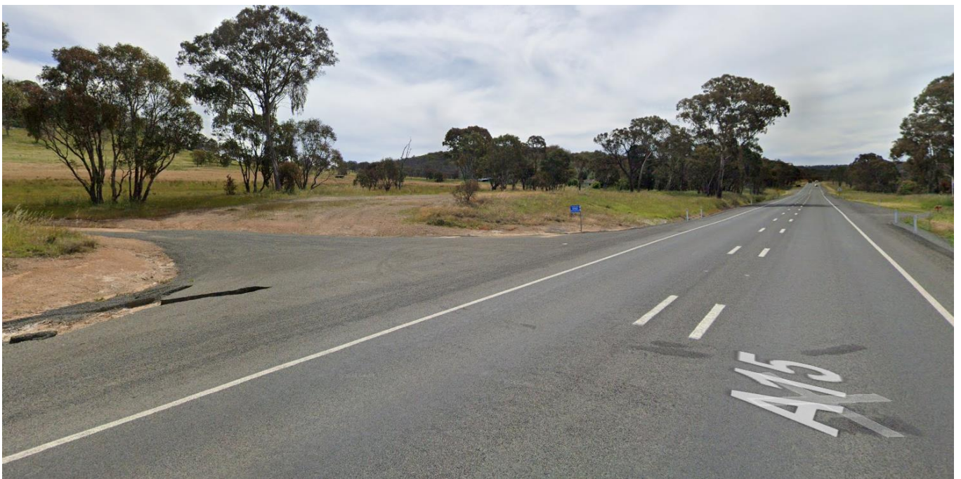
Figure 2.1 New England Highway at access road (source: Transport for NSW)
